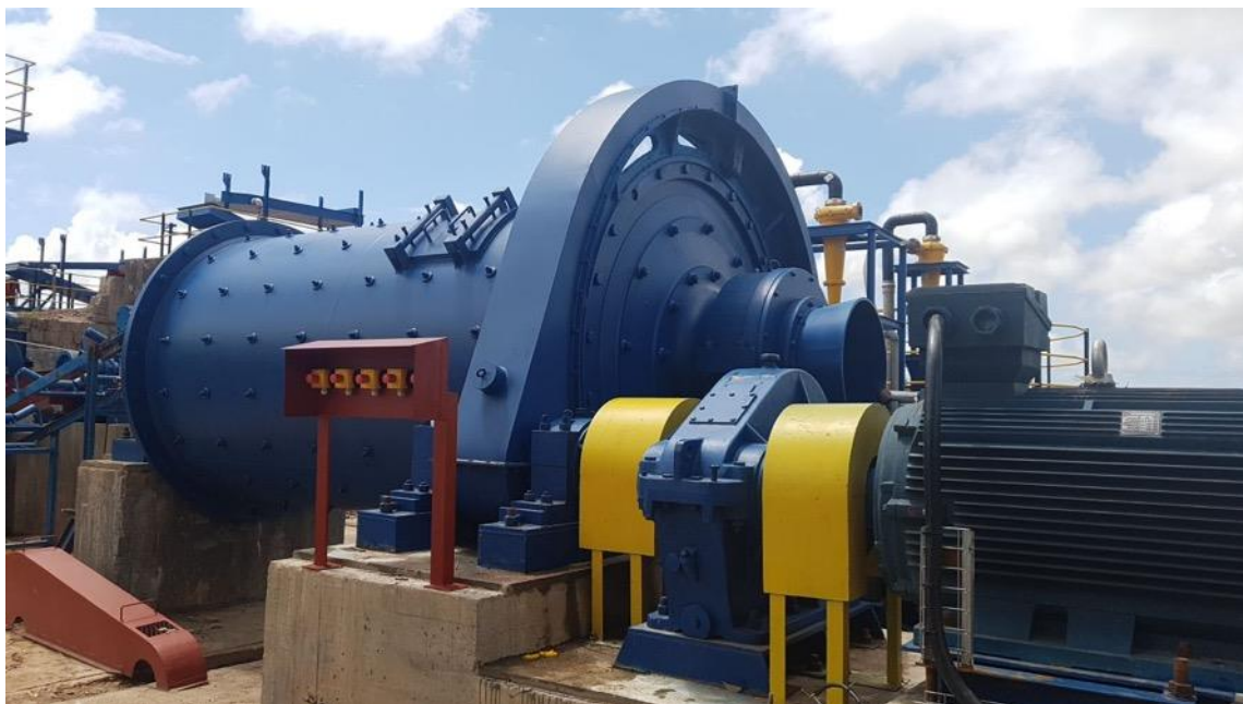
Dry commissioning of process equipment, nearing completion of Stage 1.
