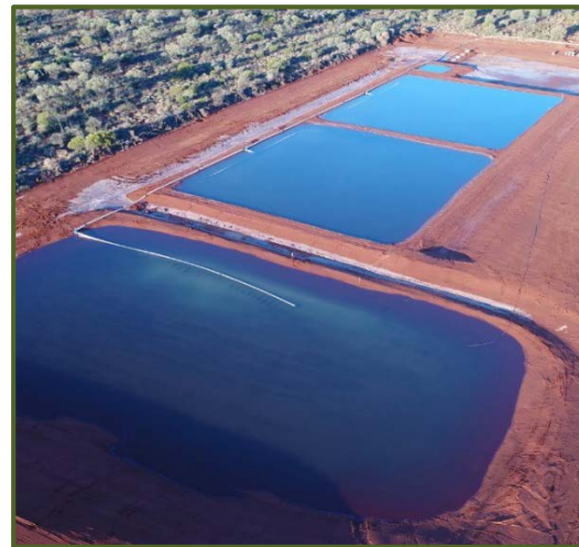
Verification Pond Trials Lined and Unlined
