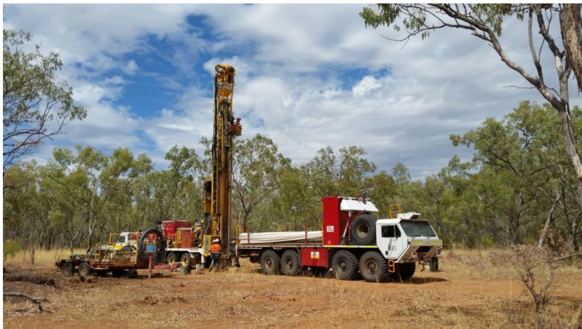
Figure 21: Groundwater monitoring bore drilling in the Lower Camp. These bores are designed to be too small to extract from and are only used to sample the quality of water for baseline environmental purposes.
