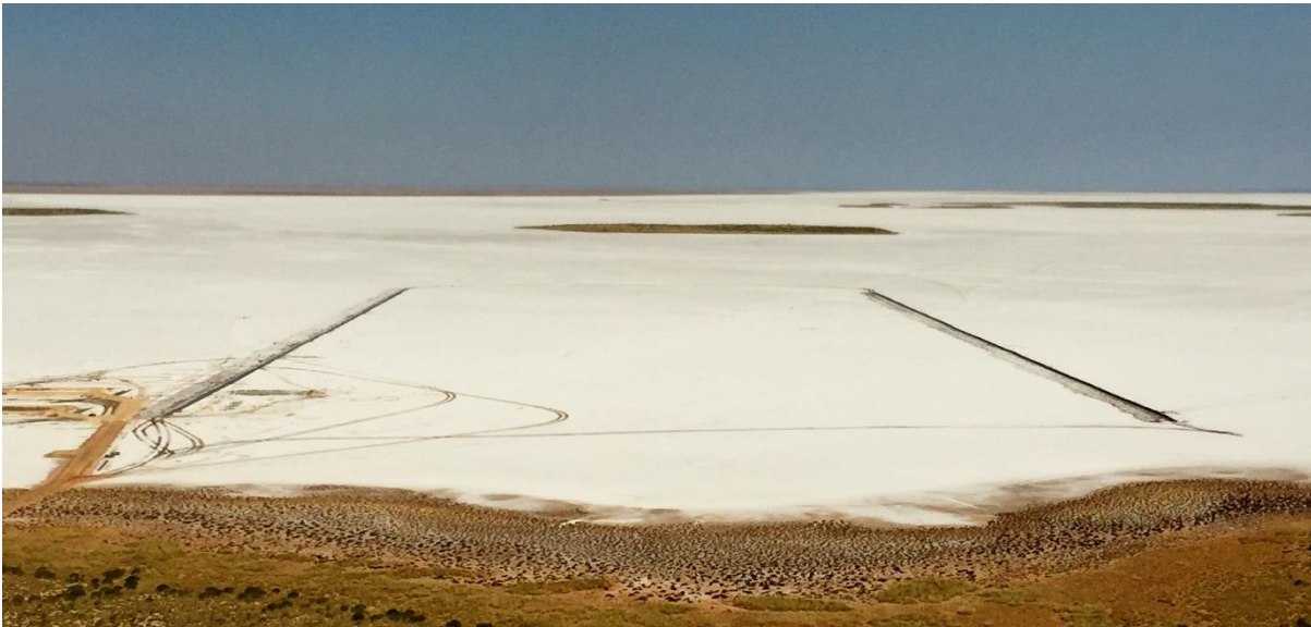
Figure 13: The Two 1-kilometre long Brine Extraction Trenches on LD
