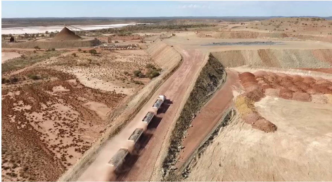
Figure 4: Road train delivering high grade ore from the Beresford underground mine at Westralia onto the ROM pad of the new 2.5Mtpa treatment plant. Note the crusher and coarse ore stockpile located to the left of the ROM pad (see Figure 3 for reference).
