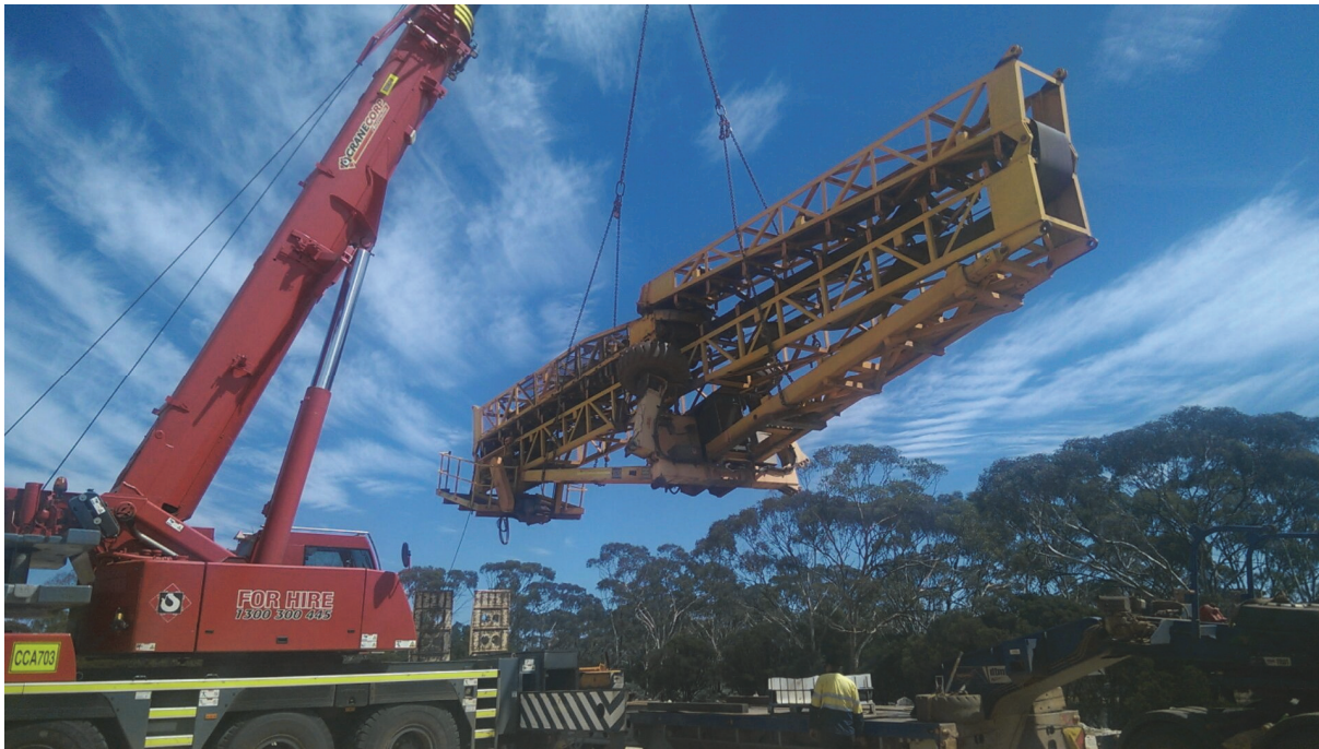
Figure 5: 22 March 2018 - Relocation of the Radial Stacker
