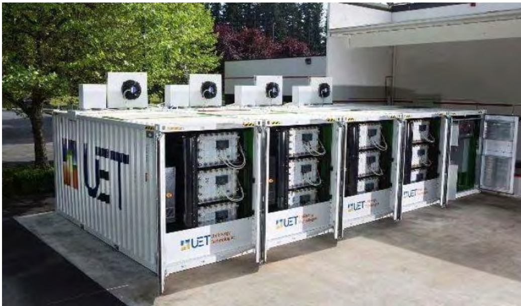
Vanadium redox flow battery storage
