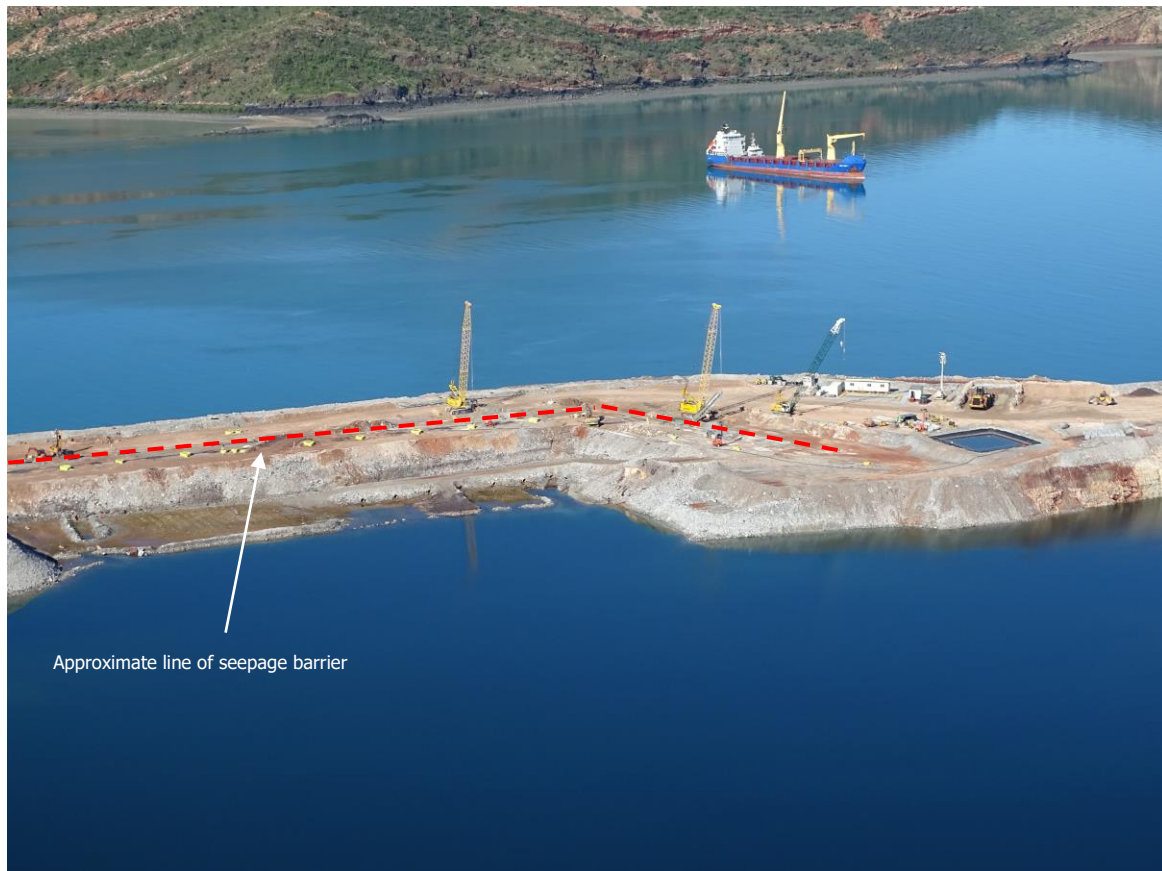
Figure 3: Seepage barrier construction, western embankment - March 2018
