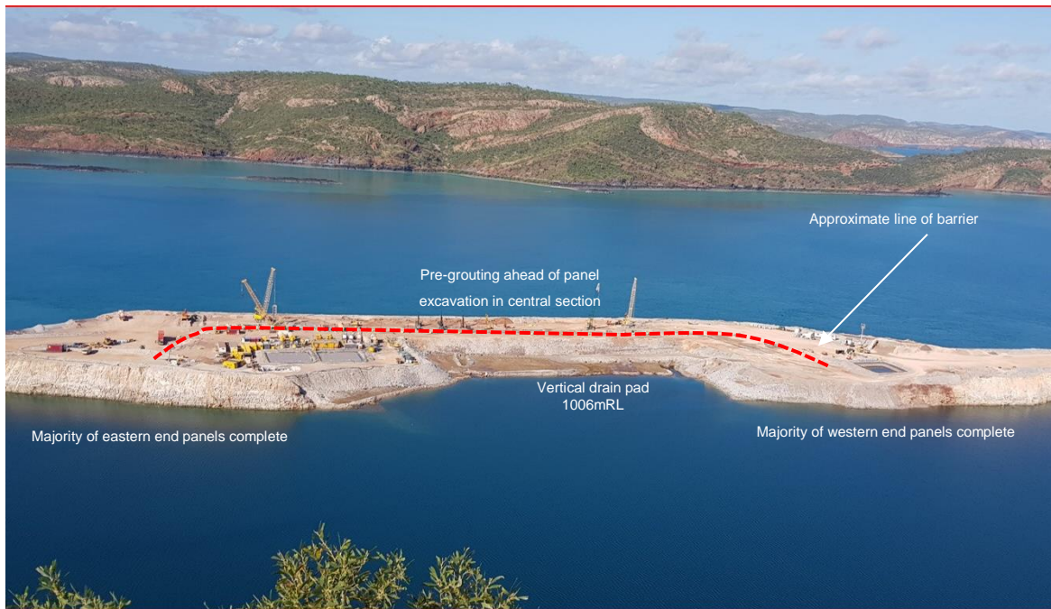
Figure 2: Seawall embankment – March 2018
