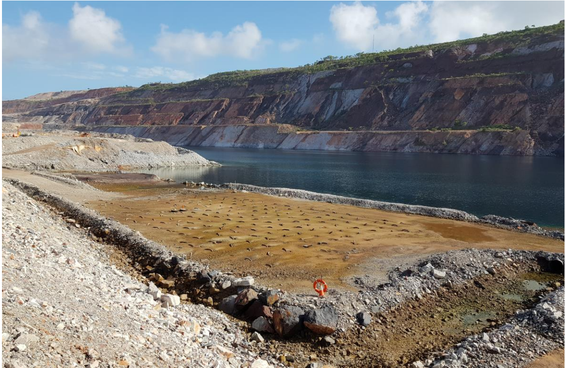
Figure 4: Vertical drain pad looking west across Main Pit to the footwall - March 2018
