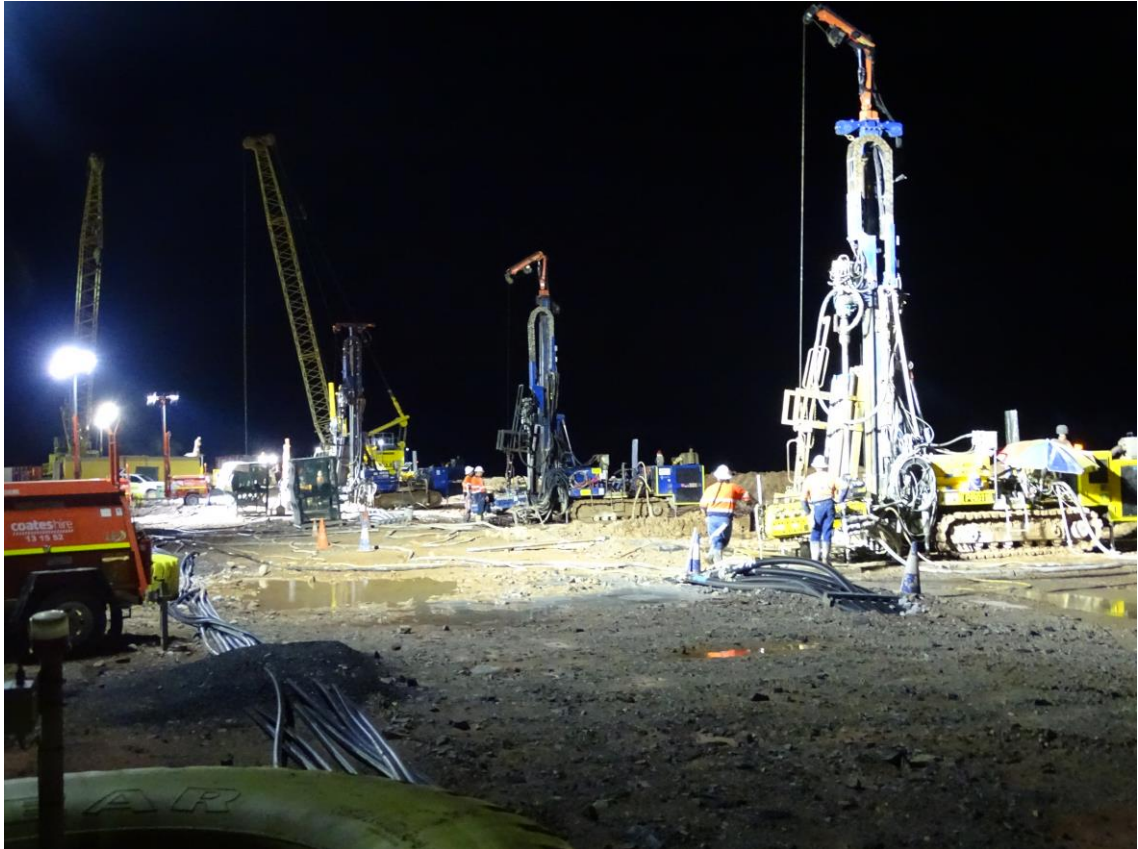
Figure 6: Grouting rigs on night shift – central embankment - March 2018
