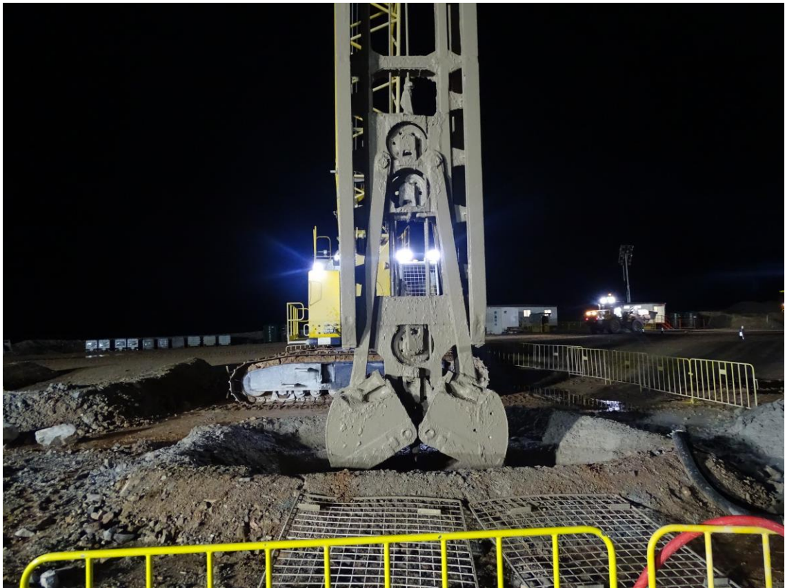
Figure 5: Panel excavation on night shift - March 2018
