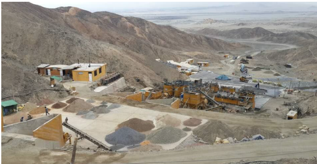
Mirador Processing Plant
