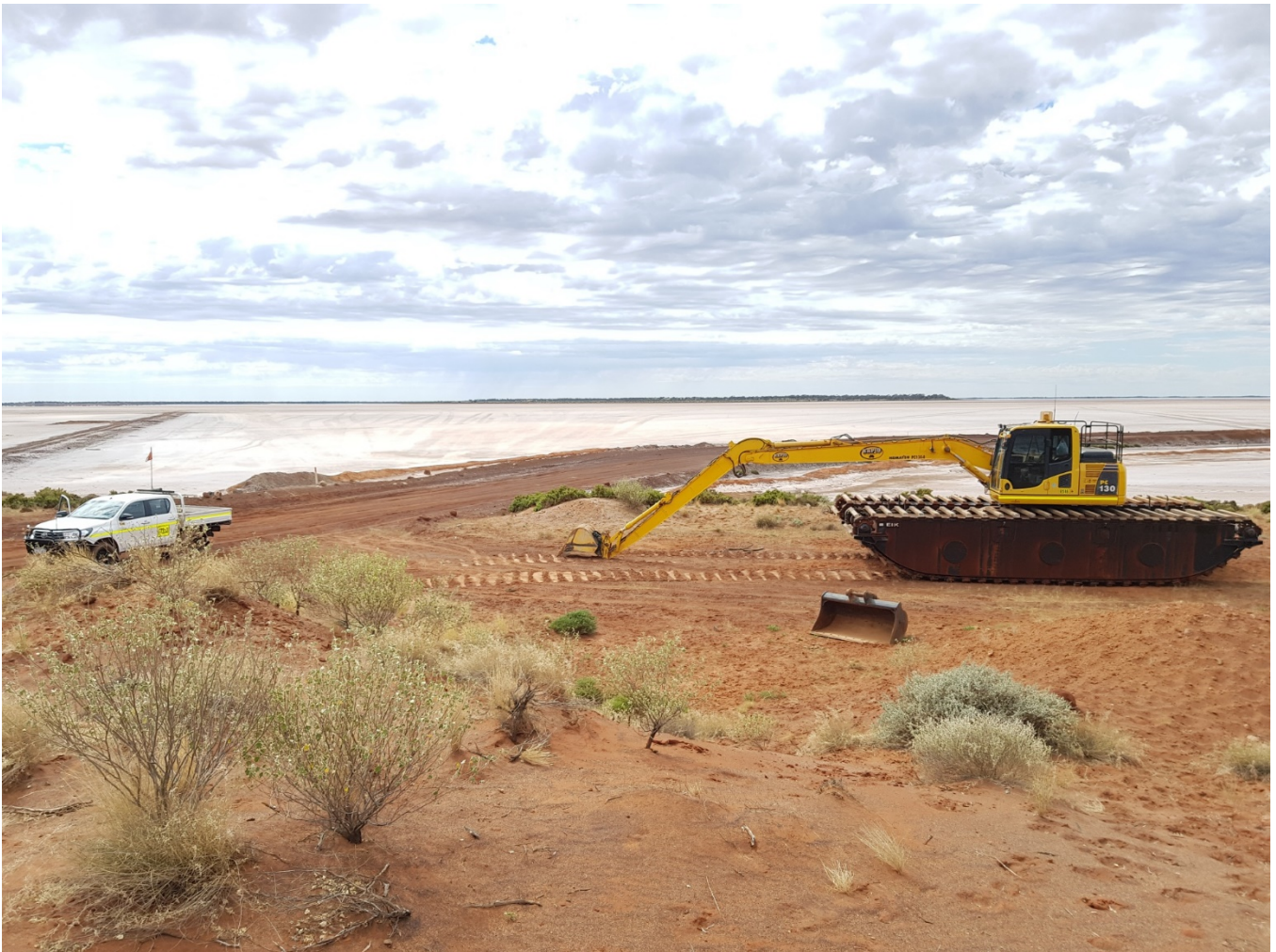
Figure 5: Amphibious Excavator on the edge of Lake Way
