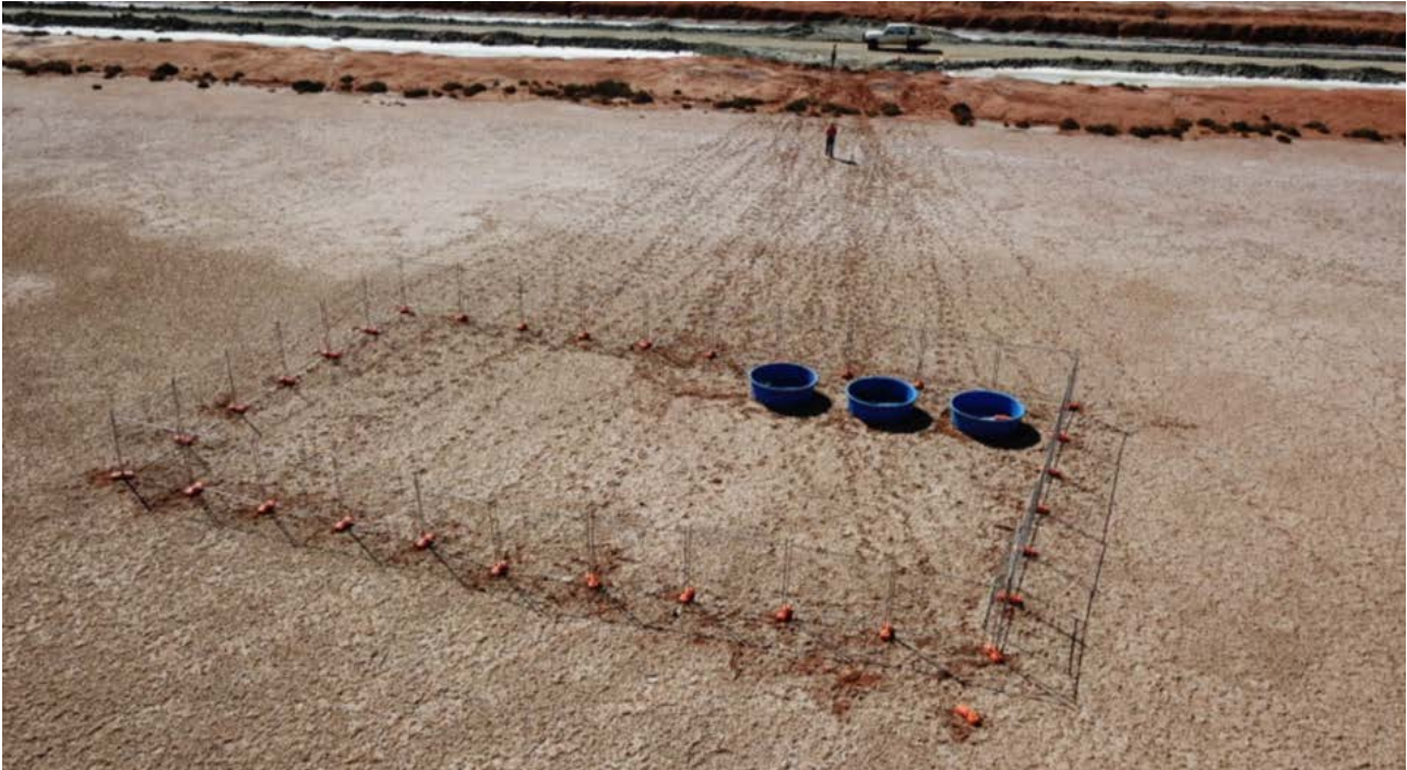
Figure 7: Lake Way SET Under Construction
