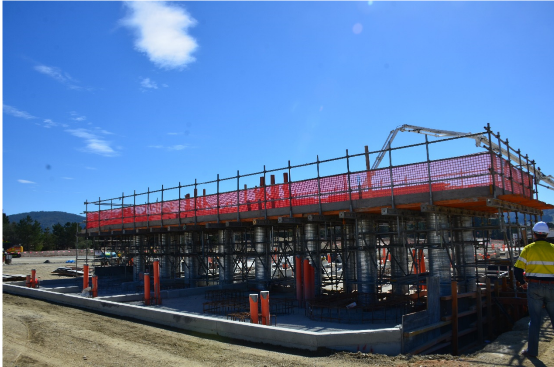
Figure 6: Float Building – preparation for pouring the float floor.
