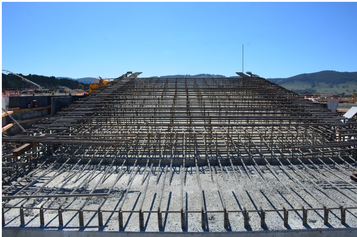
Figure 5: Steel reinforcing in place for the fine ore bin vault.
