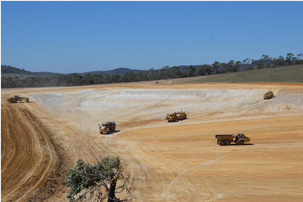
Figure 2: TSF4 dam wall construction and internal lining is well advanced.
