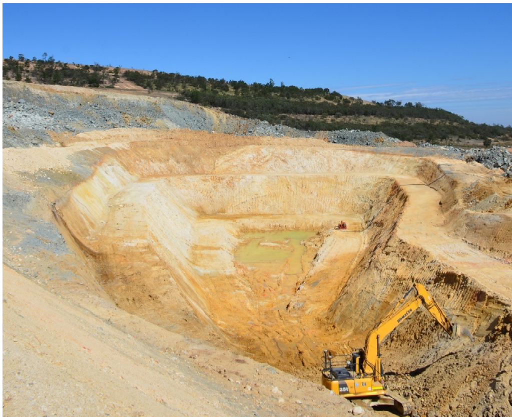
Figure 3: Box cut for underground access – last 10m bench to excavate.
