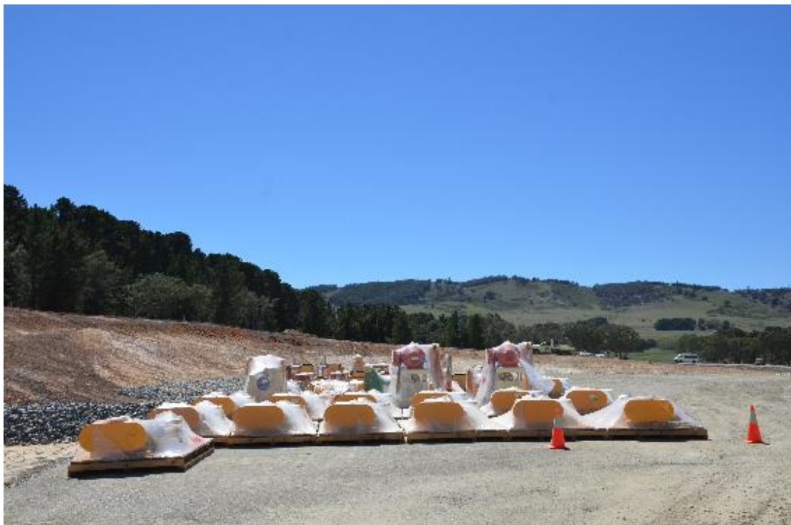
Figure 7: Arrival of the first process equipment
