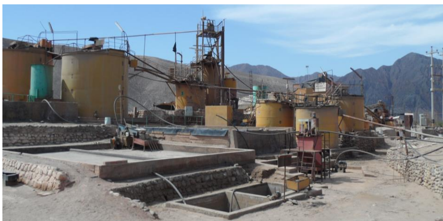
Photo 1: Tulin Gold Plant and CIL circuits
