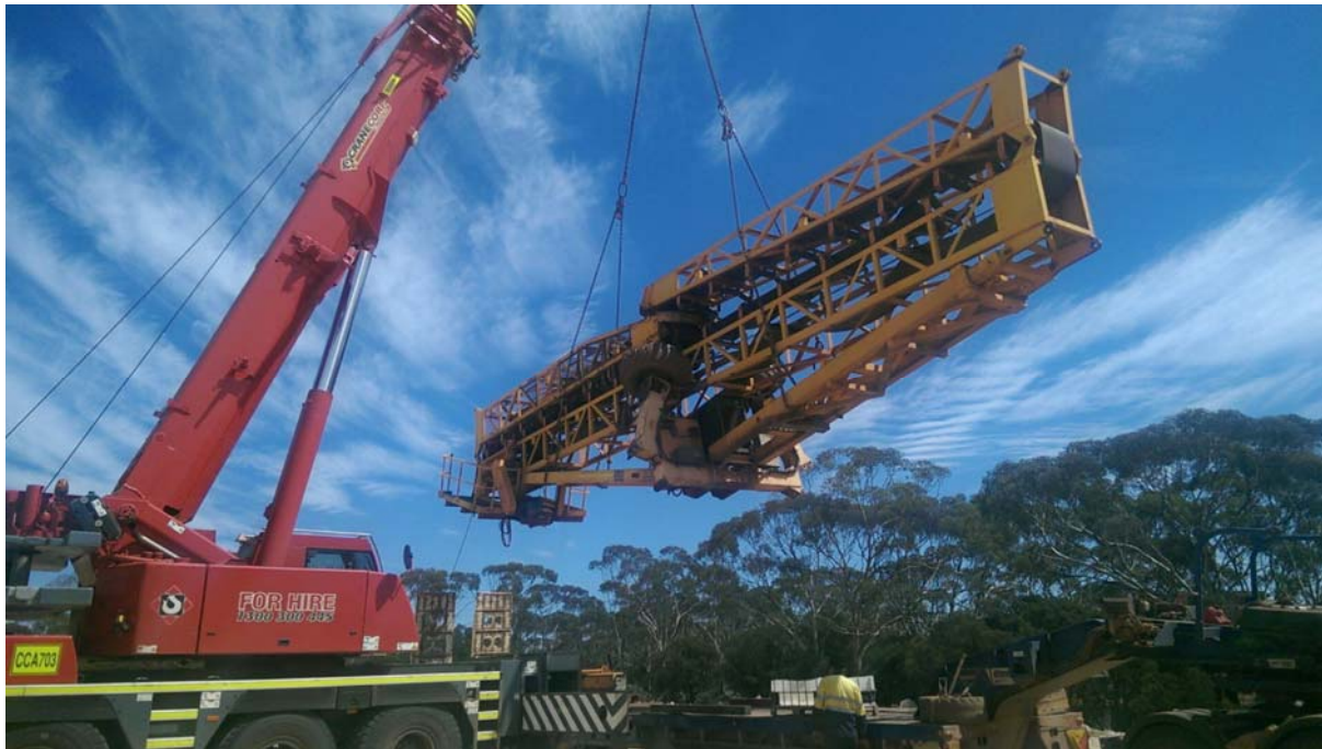
Figure 6: 22 March 2018 - Relocation of the Radial Stacker
