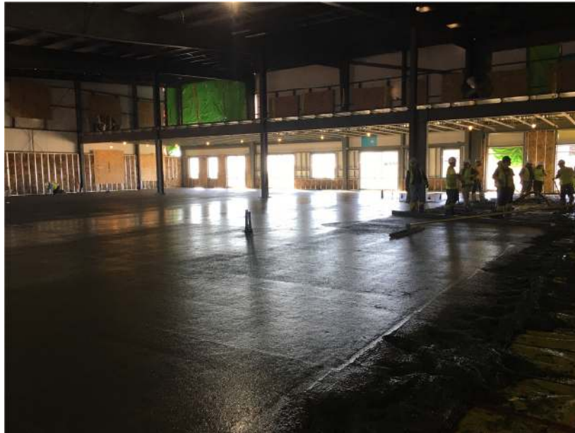
Figure 3. New factory concrete floor being poured
