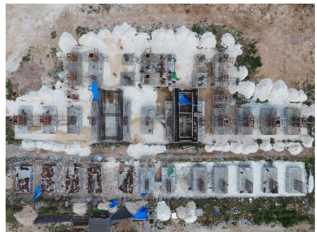
Figure 5: Aerial view of Site Foundations
