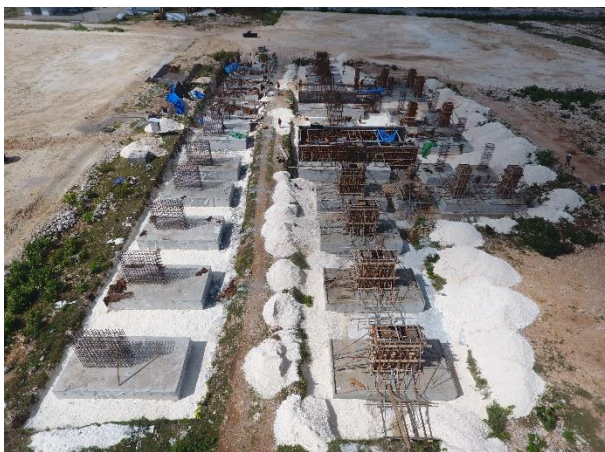
Figure 4: Site Foundations at Kupang Smelting Hub
