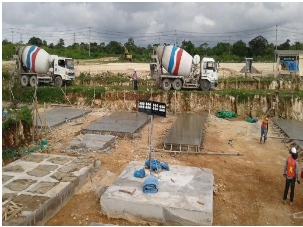
Figure 2: Concrete slabs being poured on site
