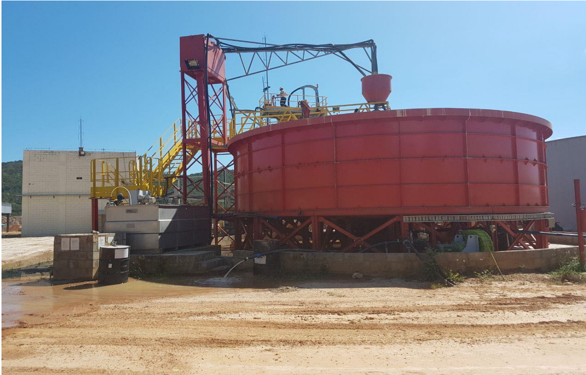
Imported thickening tank which suffered with a broken main shaft leading to 8 days downtime in March
