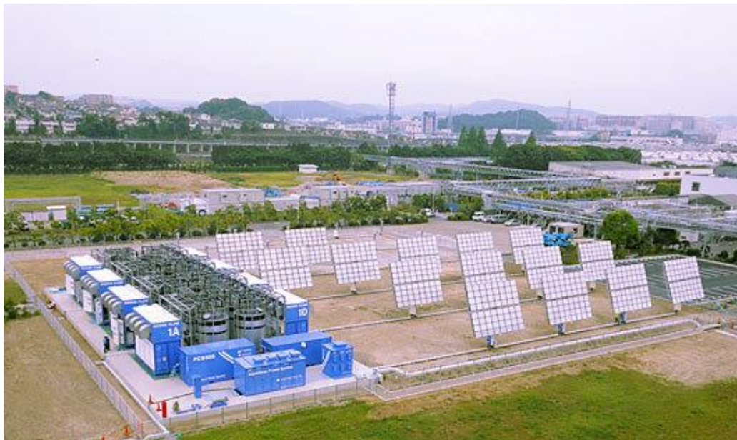
Installation of Vanadium redox flow batteries (100kWh) coupled with solar PV array (15kW) (source: VanadiumCorp.com), cost A$160,000
