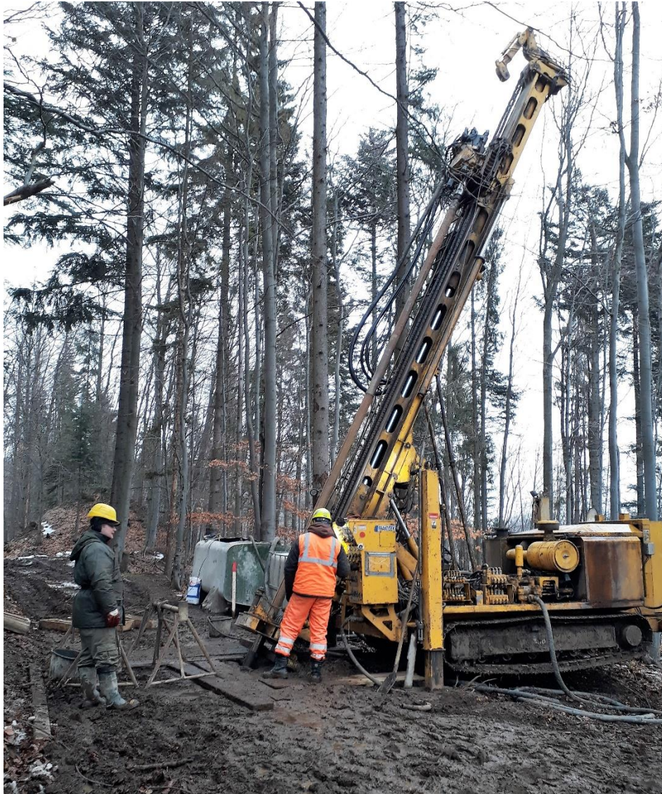
Figure 6: Commencement of Surface Diamond Drilling- Joremeny Target
