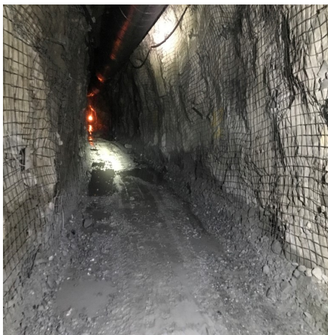
Figure 5. Backfilled ore drive
