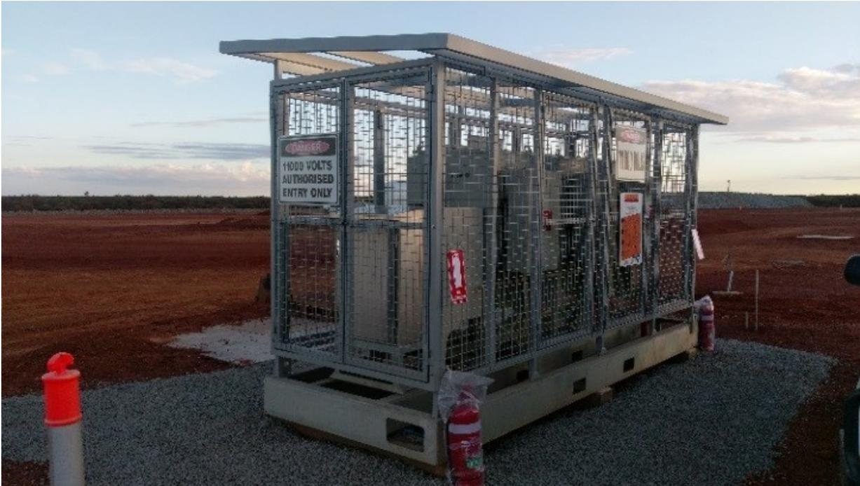
Figure 2: Monty Project: High voltage switchgear installed and ready for use
