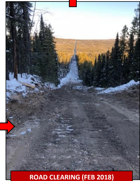
ROAD CLEARING (FEB 2018)
