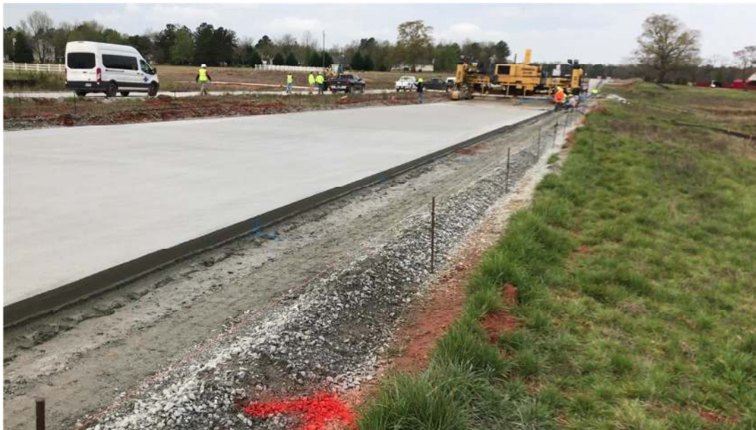
Figure 2. Completed section of highway with added EdenCrete ®
