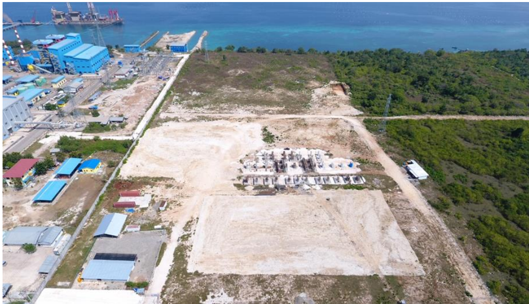
Figures 3 - Aerial overview of the Kupang Smelting Hub Facility site highlighting close proximity to power station (top left)
