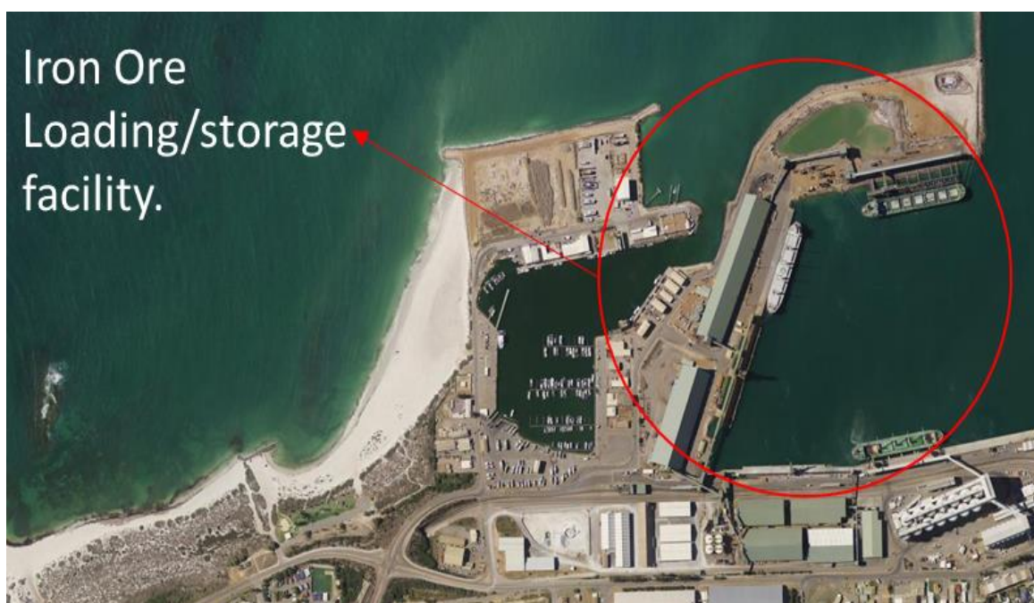
Figure 3 Iron Ore loading and storage facilities at Geraldton port
