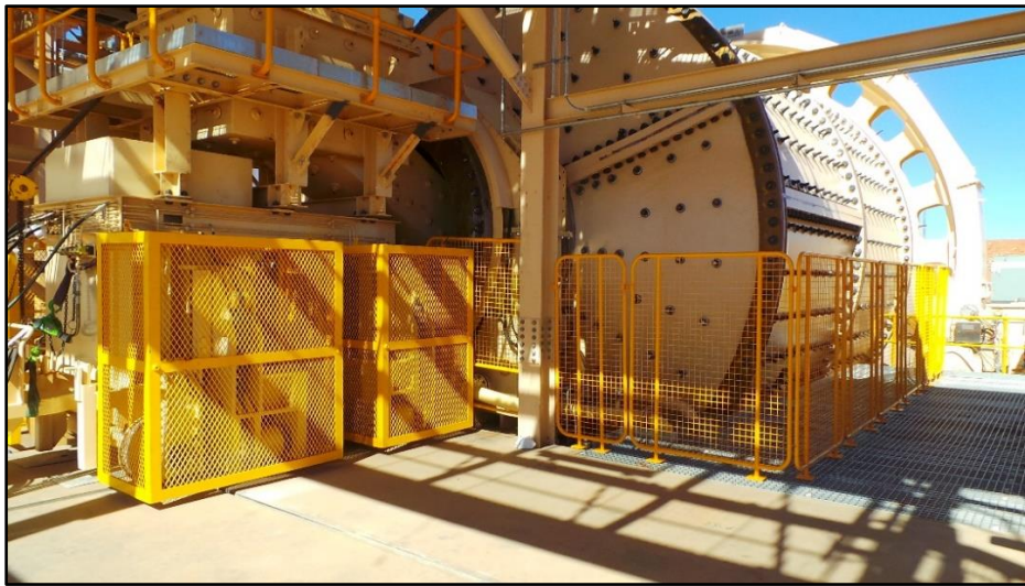
Photo 5: SAG Mill Installation Complete with Ore Commissioning Underway
