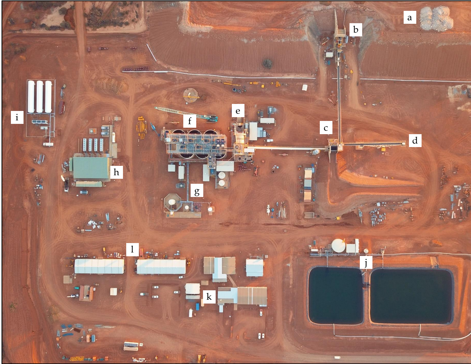
Photo 3: Dalganga Process Plant Site Overview
