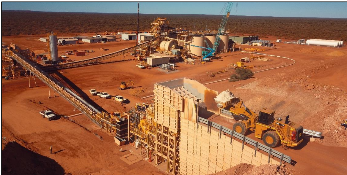
First Ore fed into the Primary Crusher
