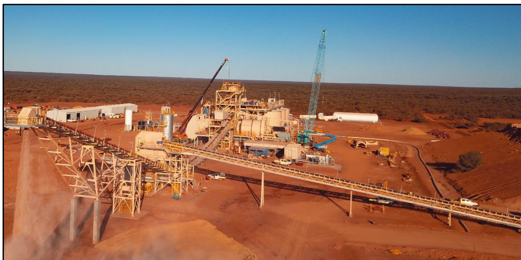
Photo 2: Dalgaranga Plant Ore Commissioning underway
