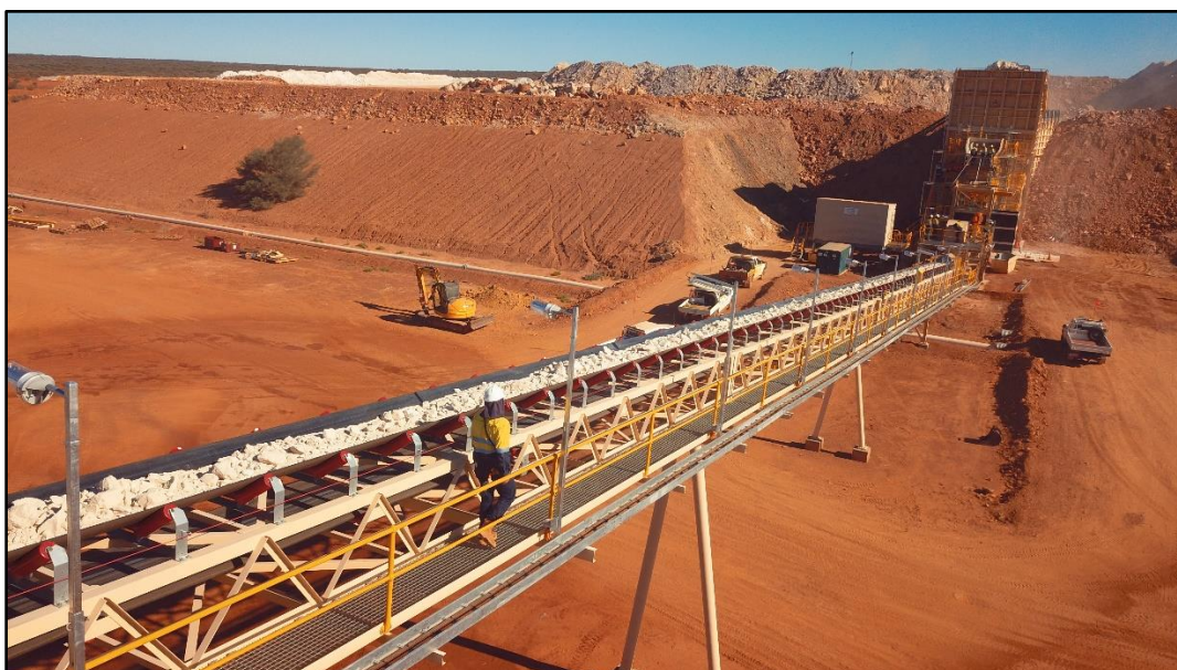
Photo 1: Dalgaranga Plant Ore Commissioning underway
