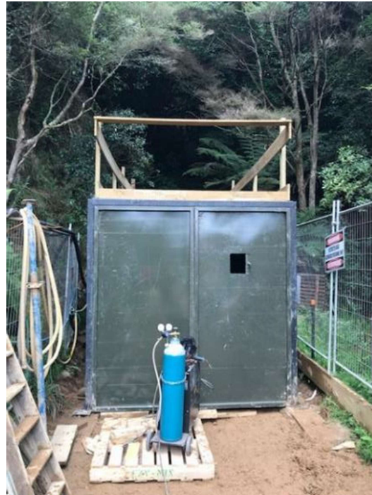
Figure 2 - Completed ventilation lock at No 8 Level Portal
