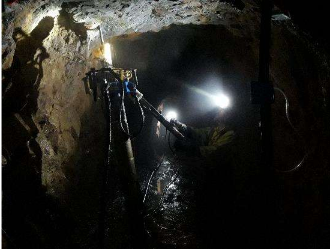
Figure 3 - installation of rock bolts in Keillors Crosscut
