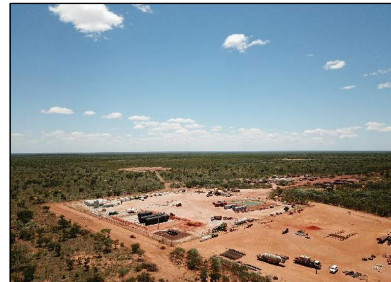
Ungani field facility
