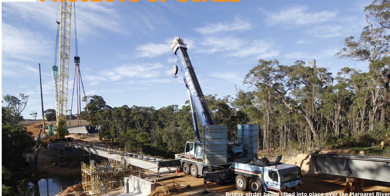
Bridge girder being lifted into place over the Margaret River
