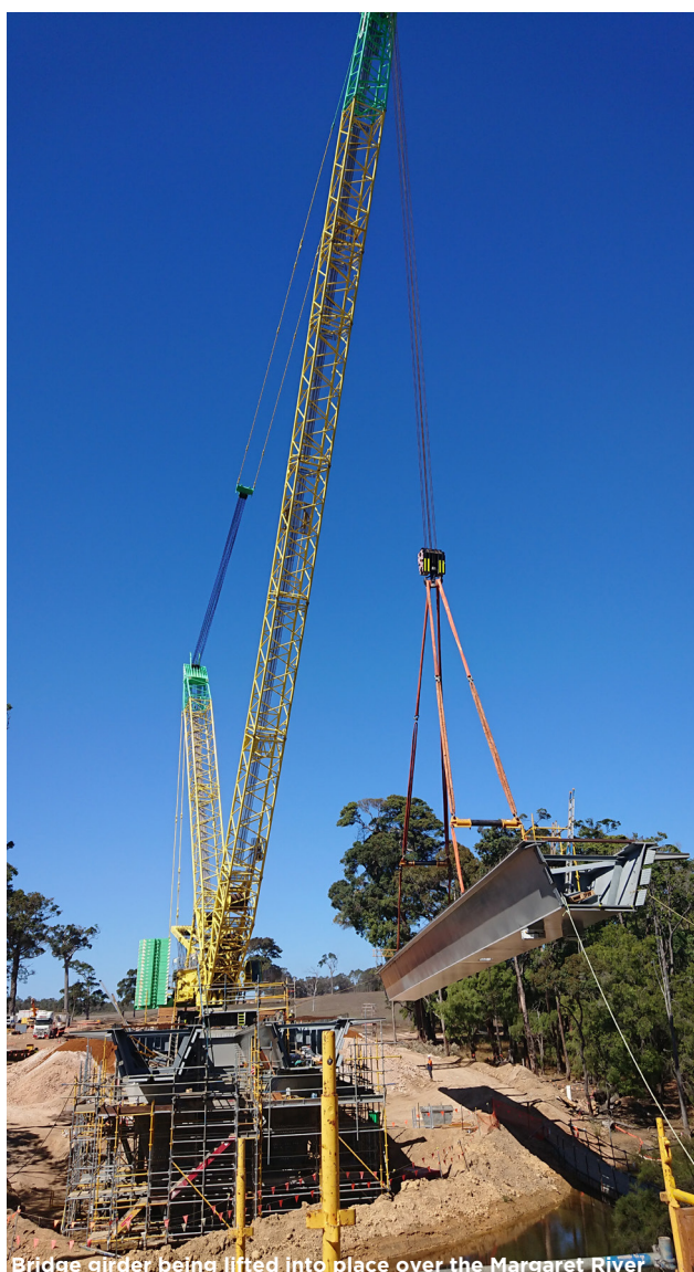
Bridge girder being lifted into place over the Margaret River
