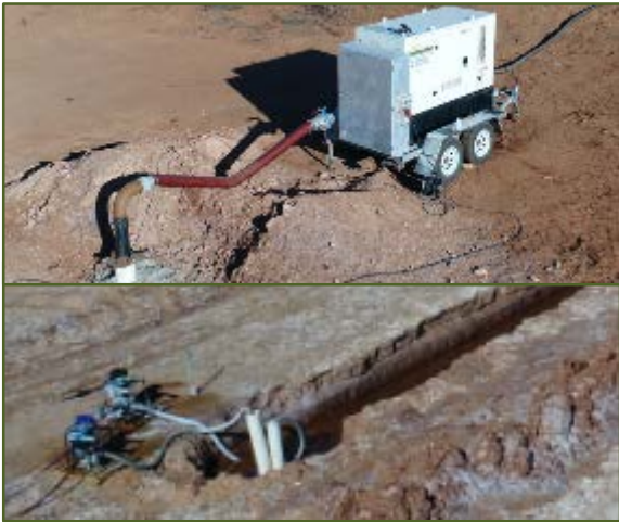
Brine Pumping from Bores and Trenches >175 Million litres successfully pumped to date
