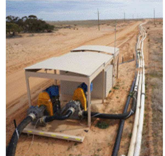
Slurry Booster Stations & pipelines
