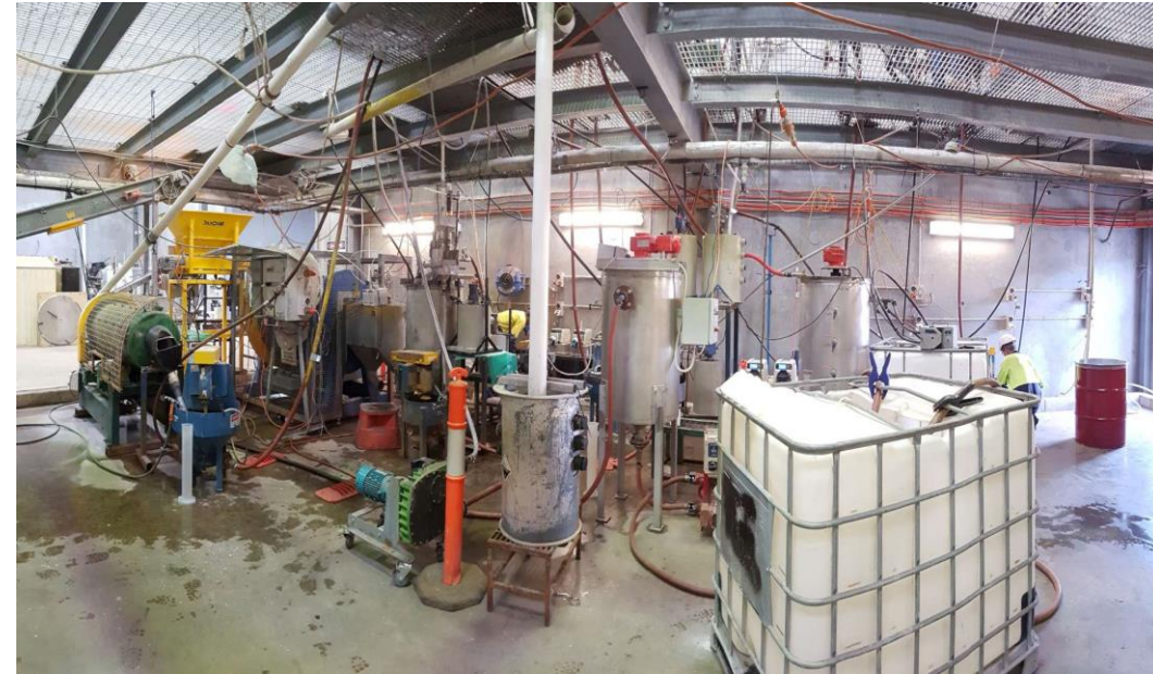
Flotation Pilot Plant - Milling, Conditioning, De-sliming and Reagents
