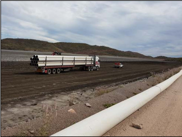
Figures 5 & 6: Delivery and installation of tailings transfer pipework to transport slurry to the Processing Plant
