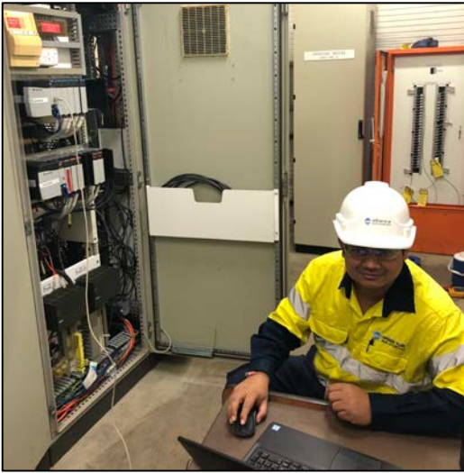
Figures 15 & 16: Plant control system installation and point-to-point testing underway (left) and sand blasting and repainting of thickeners prior to water commissioning activities (right)
