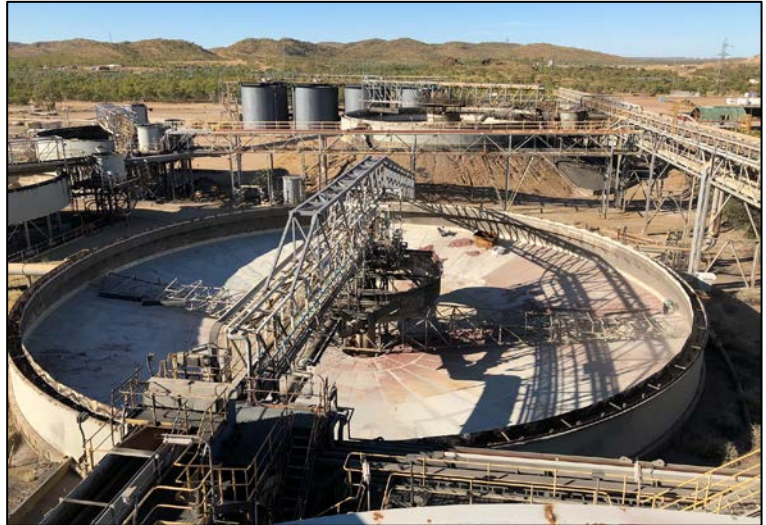
Figures 15 & 16: Plant control system installation and point-to-point testing underway (left) and sand blasting and repainting of thickeners prior to water commissioning activities (right)
