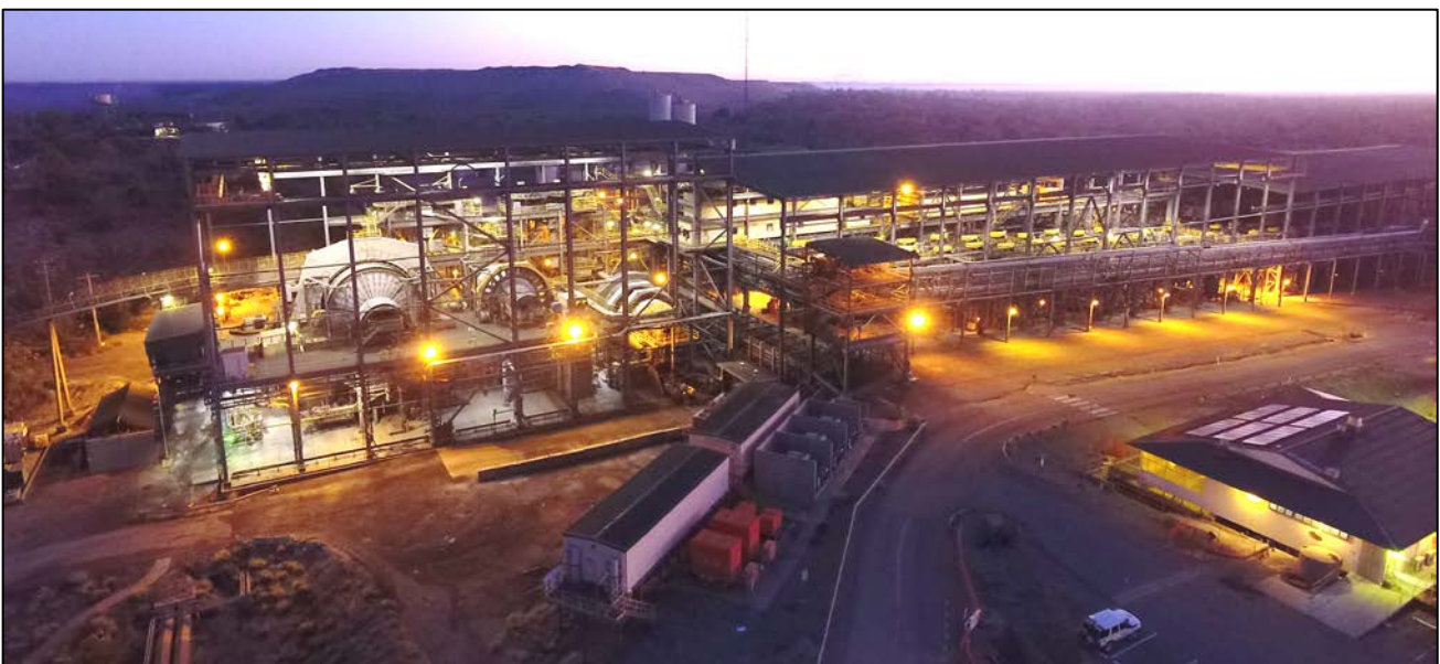
Figure 1: Century Processing Plant refurbishment well advanced with commissioning due in July 2018
