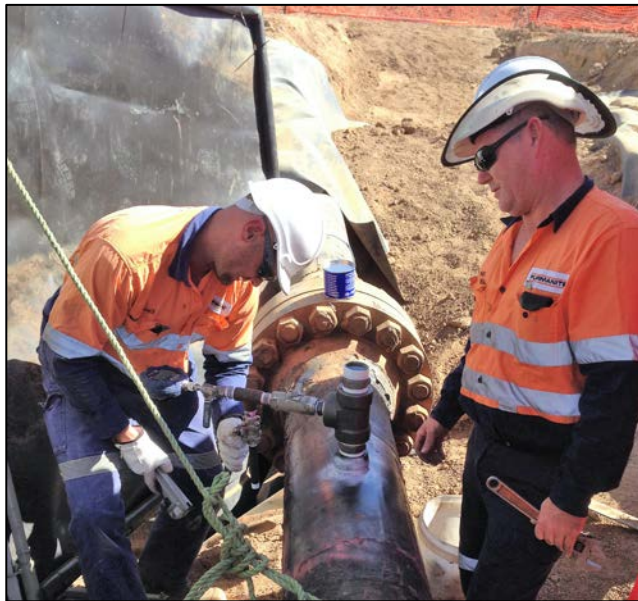
Figures 21 & 22: Initial pipeline 'hot tapping' for localised draining, controlled removal and capture of water (left) and Process Plant & Pipeline Superintendent Chris Portelli with the extracted cleaning pig (right), allowing for water commissioning activities to begin in June
