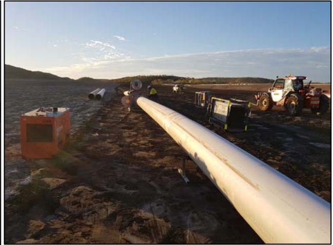
Figures 5 & 6: Delivery and installation of tailings transfer pipework to transport slurry to the Processing Plant
