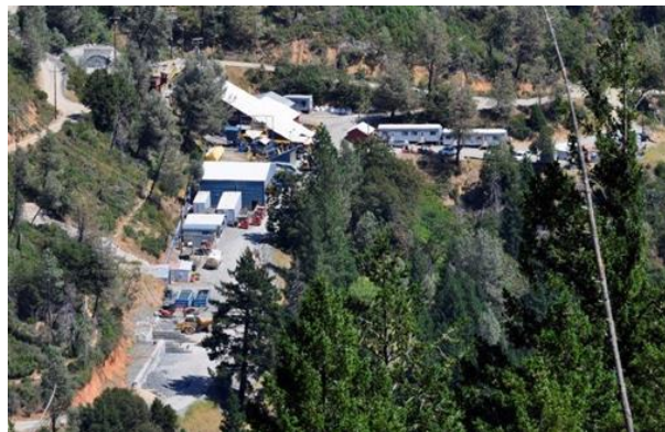
Figure 4: Aerial view over mine infrastructure
