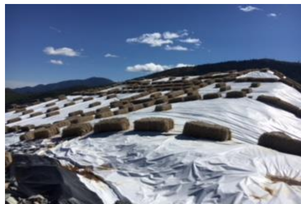
Figure 8: Dry tails stack
