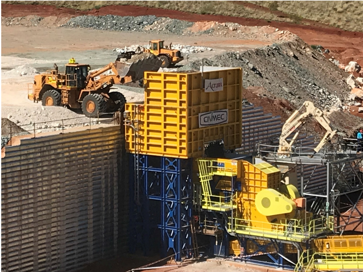
Operations continue to ramp up ahead of first product sales
