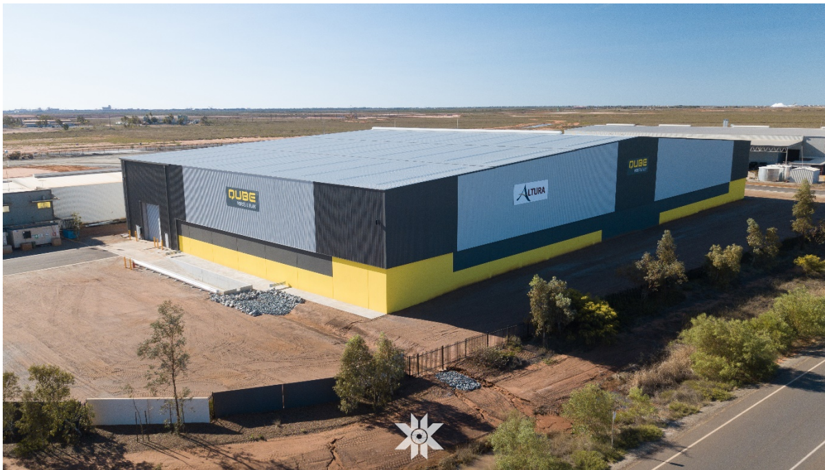
The completed product storage shed located in Port Hedland
