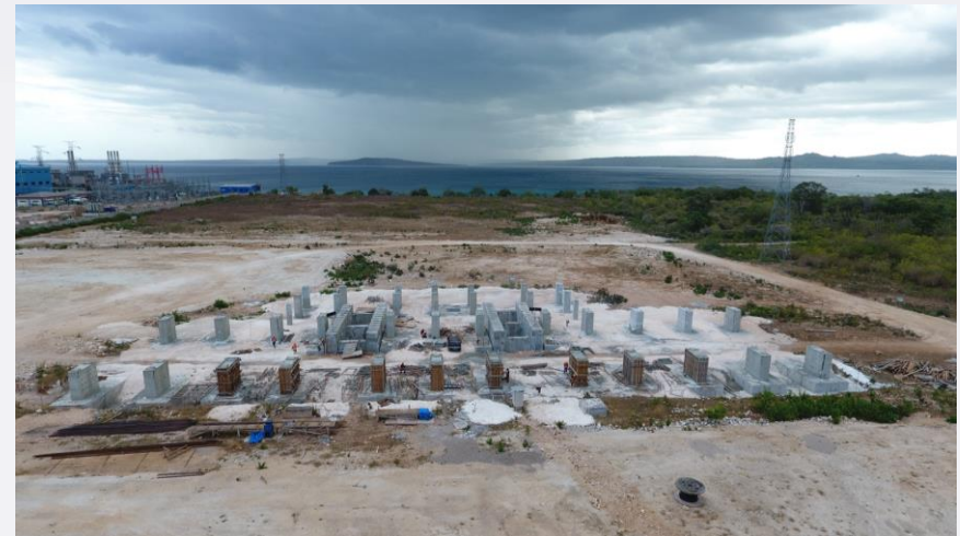
Figure 3: Concrete Foundations Finished at Smelting Hub Facility
