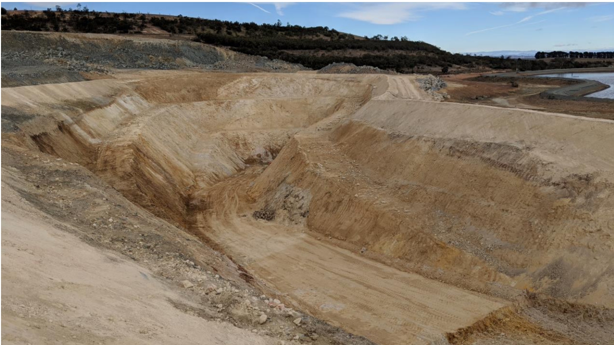
Figure 9: Box cut excavation complete
