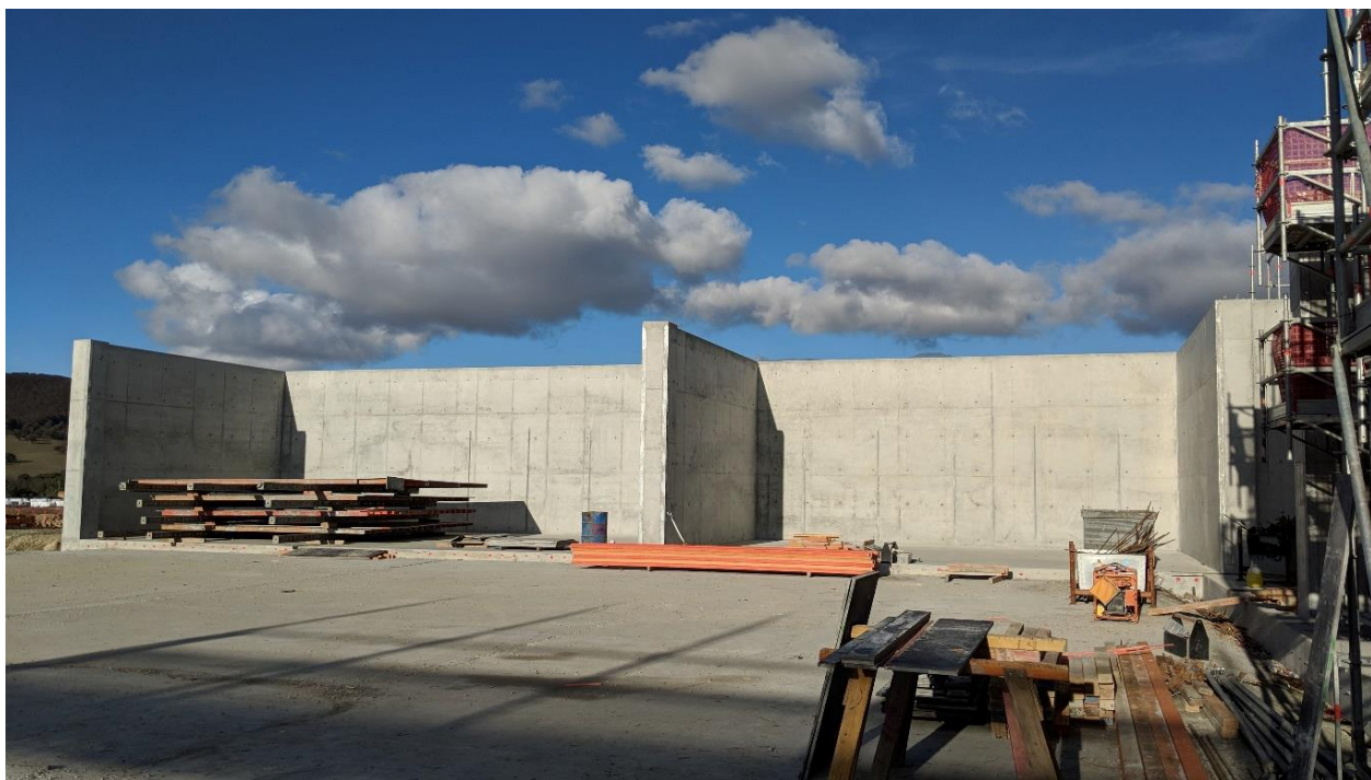
Figure 3: Copper and lead concentrate storage bays
