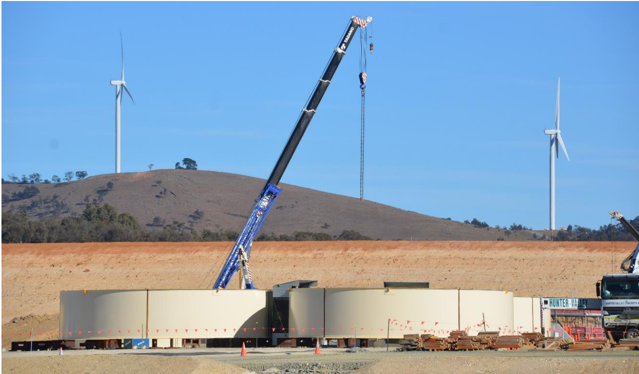
Figure 6: Processing plant feed surge tank being erected
