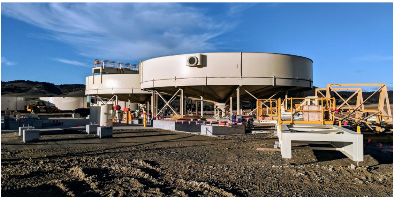
Figure 7: Final tails and reclaimed tailings ore feed thickeners installed
