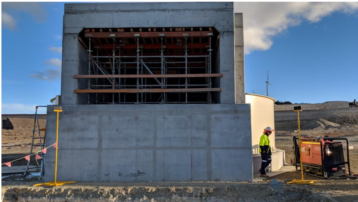
Figure 2: Fine ore bin foundations and feeder vault ("the bunker")
