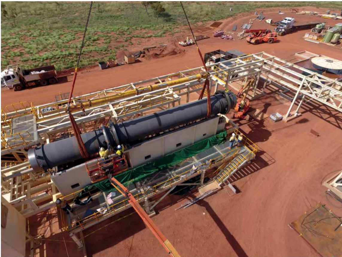
FIGURE 3.1: BROWNS RANGE – HEAVY RARE EARTHS CONCENTRATOR – ROTARY KILN INSTALLATION
