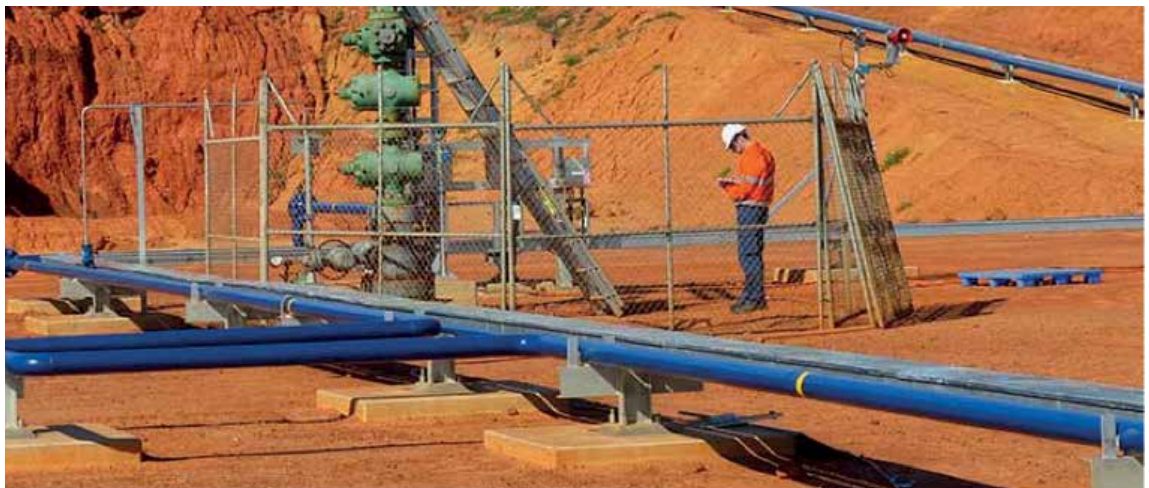
FIGURE 3.7: RED GULLY GAS AND CONDENSATE PROCESSING FACILITY – WELL HEAD
