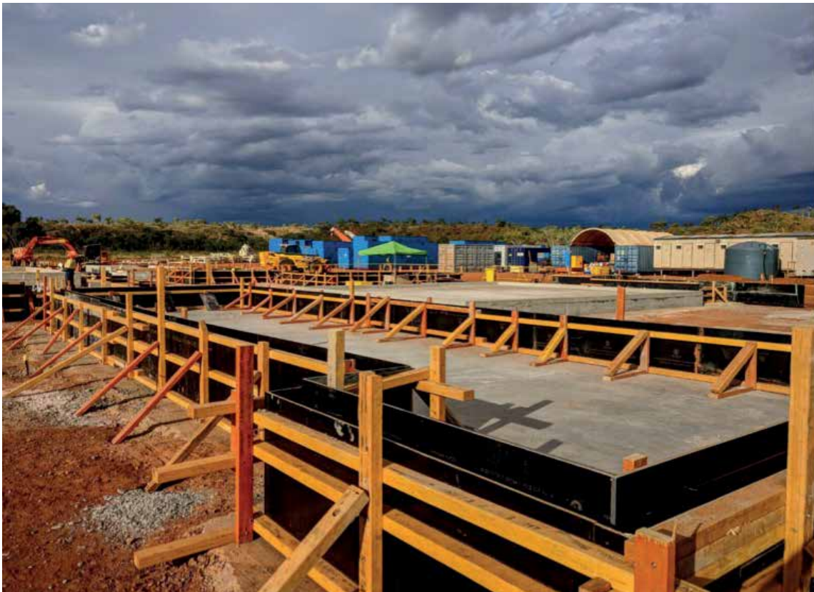
FIGURE 3.4: BROWNS RANGE – HEAVY RARE EARTHS PROCESSING FACILITY – CONCRETE INSTALLATION
