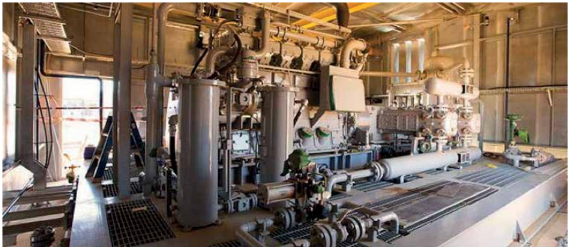
FIGURE 3.5: RED GULLY – GAS AND CONDENSATE PROCESSING FACILITY – GAS EXPORT COMPRESSOR
