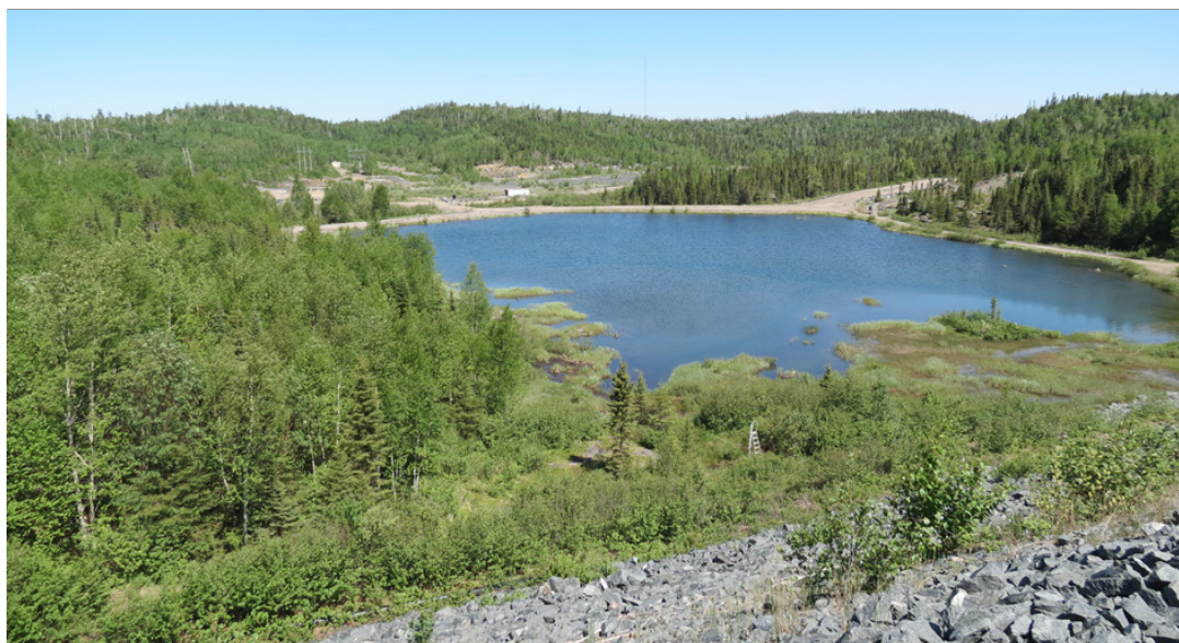
Figure 12 – View from Tails Storage Facility to Old Plant Site (Superior 2018)
