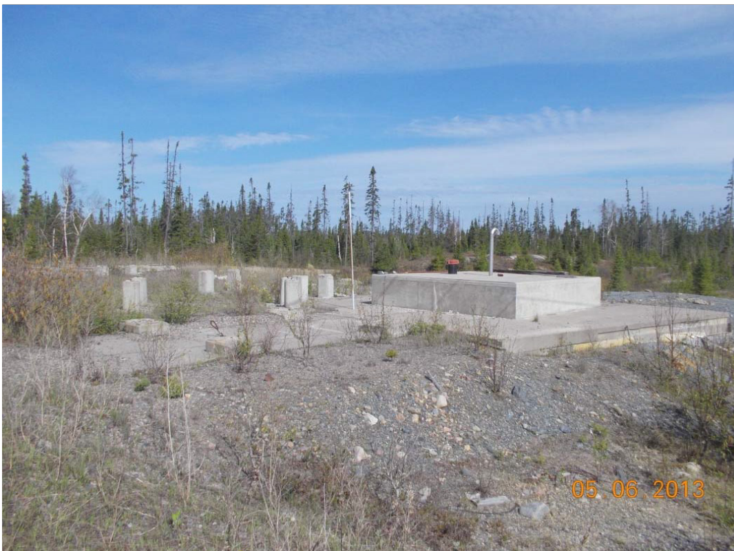
Figure 3 – Capped Ventilation Shaft at Project Site (Silvore Fox 2013)
