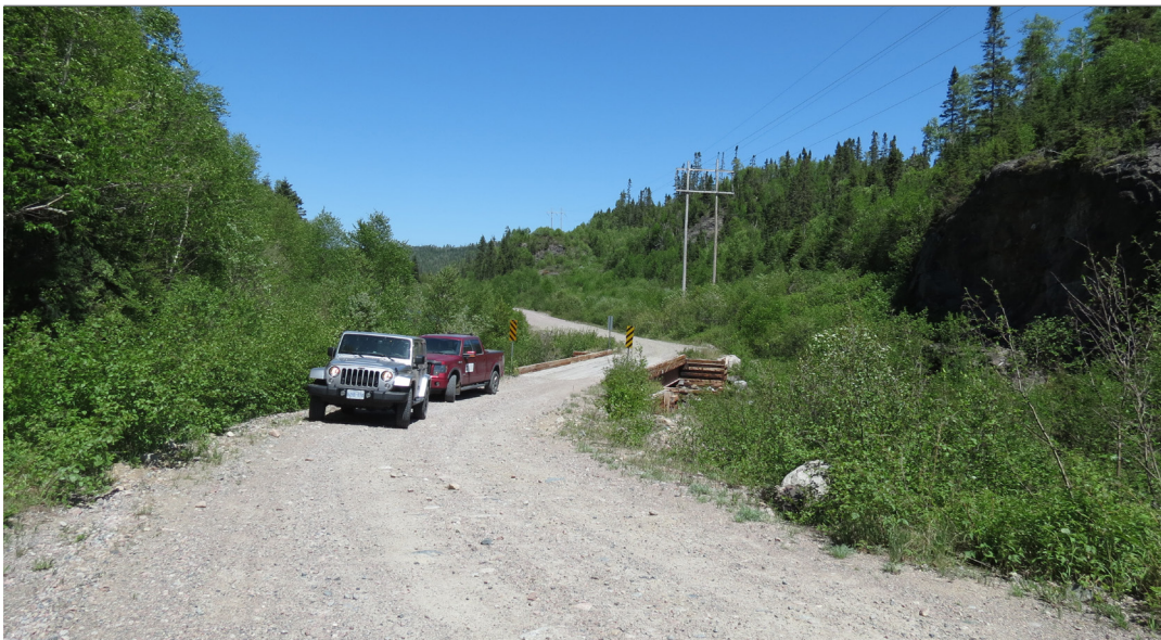
Figure 6 – Project All Weather Access Road with Main Power (Superior 2018)
