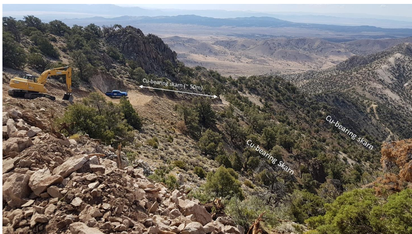
Figure 1: Roadworks and drill pads nearing completion. At least seven drill holes for up to 3000m are planned from drill pads HIP002-HIP004 along the Upper Accrington road as part of an overall 7000m program.
