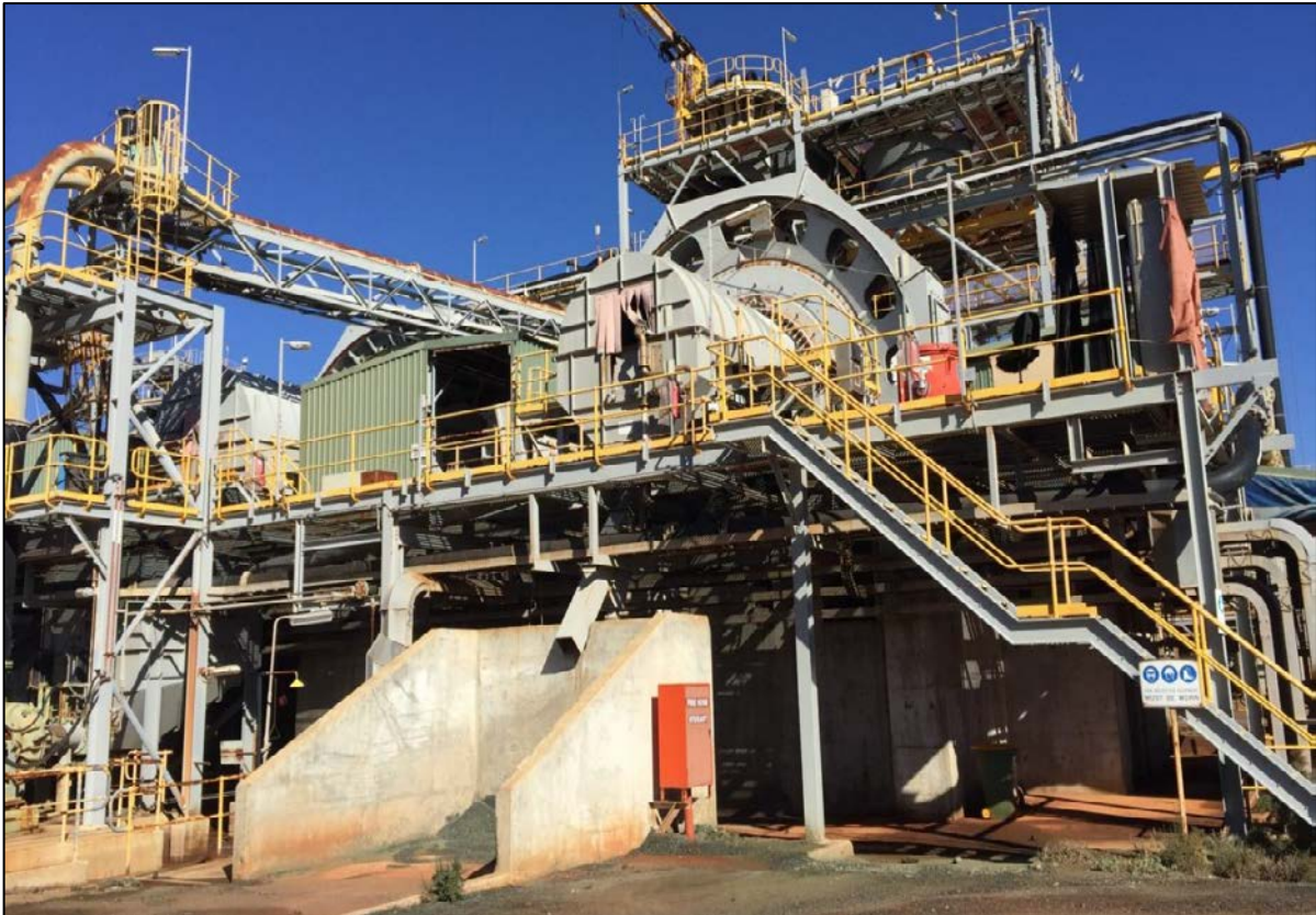
Figure 2: Black Swan Process Plant
