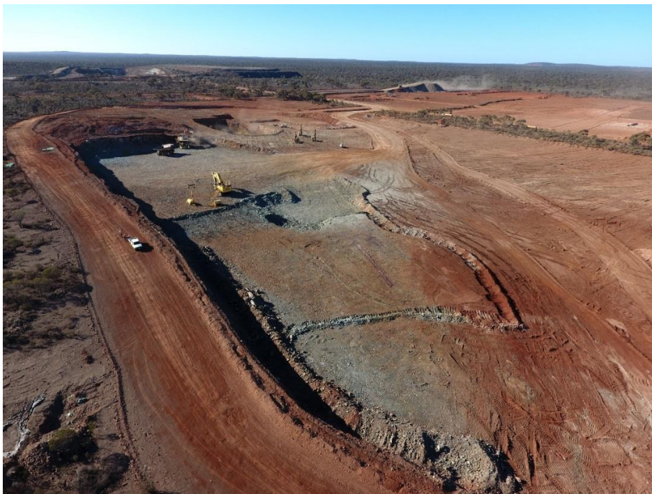
Figure 1: Overburden and stripping underway at Aldiss
