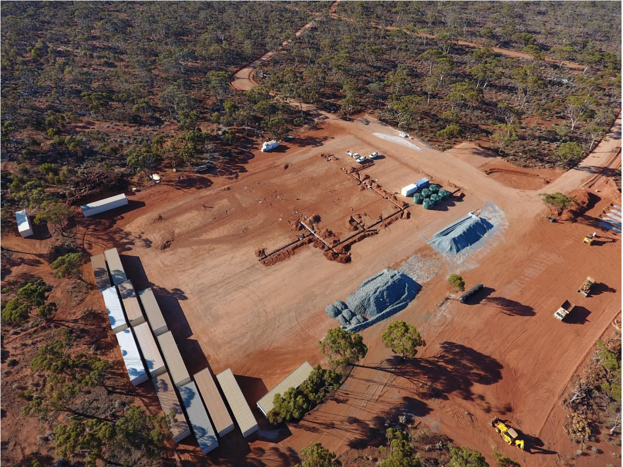
Figure 2: Accommodation camp construction at the Aldiss Mining Centre
