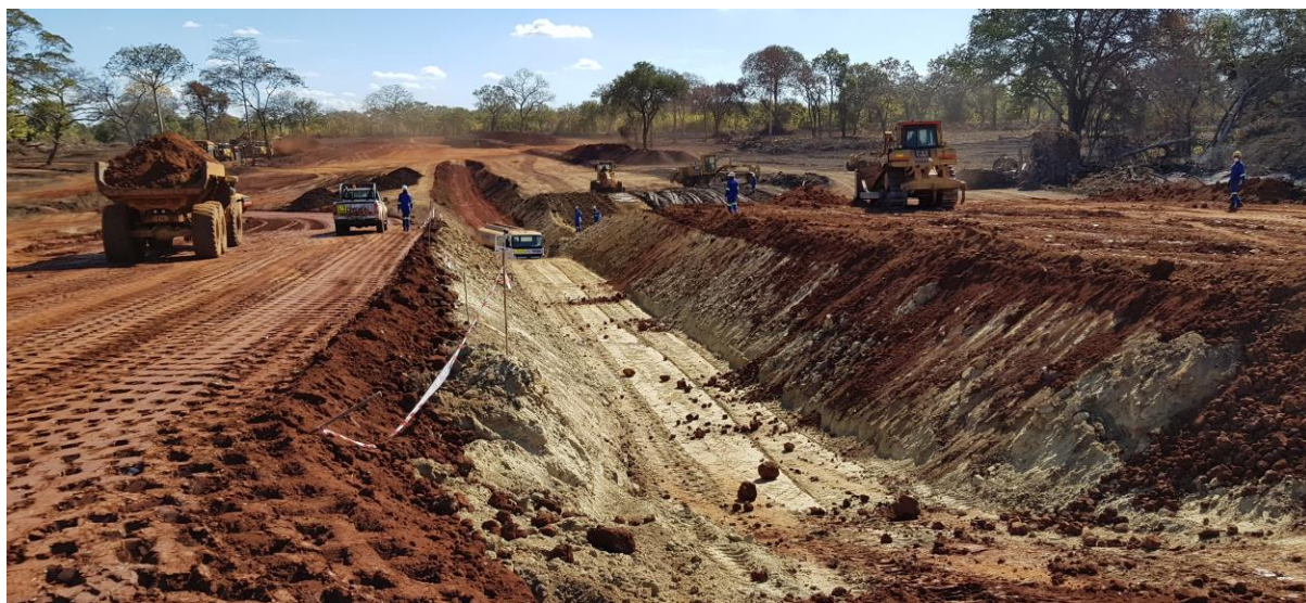
Figure 3. Montepuez Graphite Project Tails storage facility under construction, due for completion in October.
