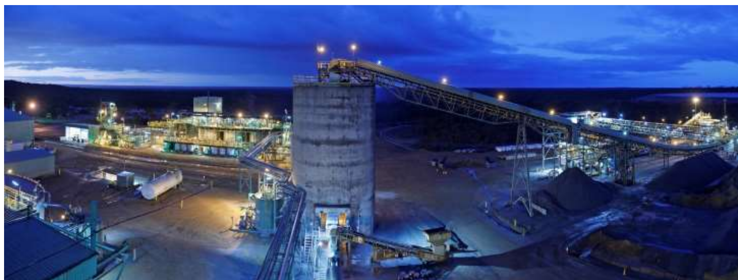
Panorama of Cosmic Boy mill and the new MREP facility
