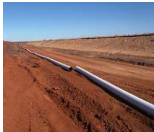
HDPE pipe ready to weld along existing ponds
