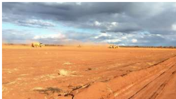
Scrapers operating in WMP 8
