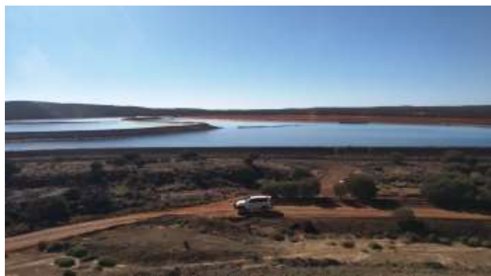
WMP 6 and 7 in foreground with WMP 8 cleared in the background
