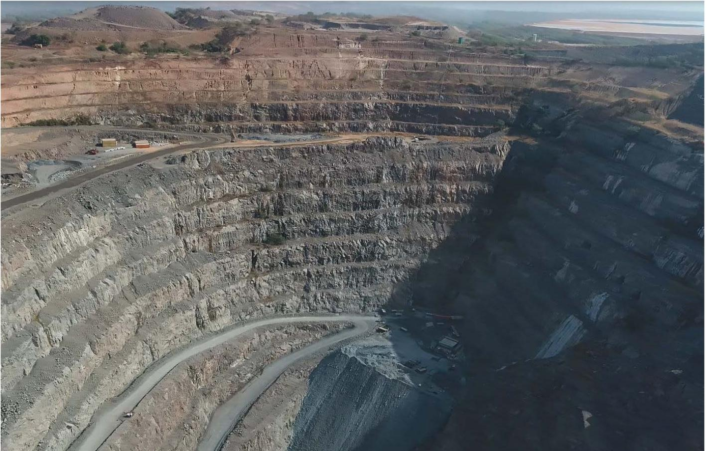
**Figure 4: Syama Open Pit with 1,200mRL mid-pit portal in centre right of photo**
