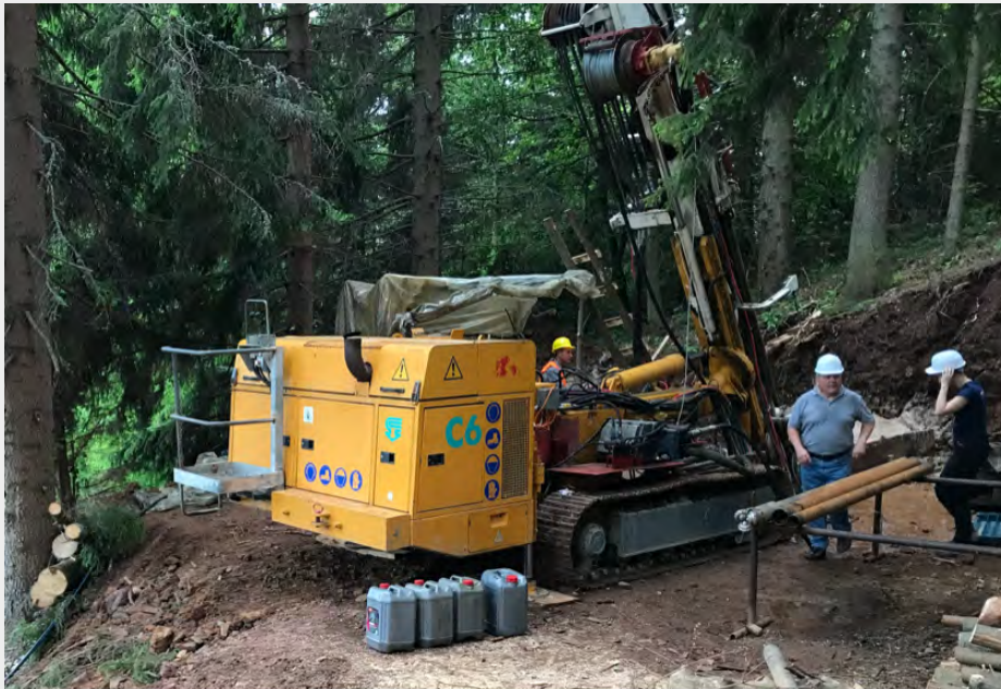
Drill rig onsite at Brestic Jurasevac
