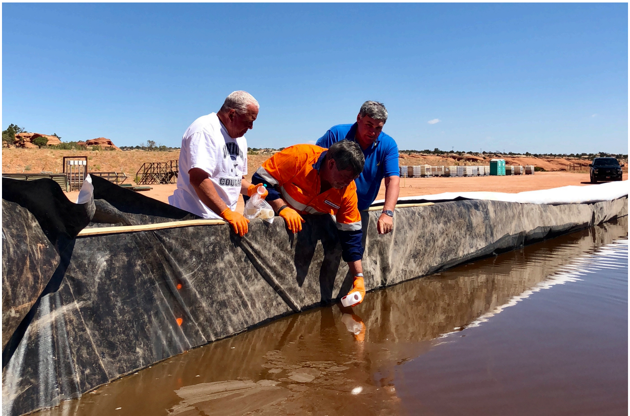
Figure 1 On-site test evaporation ponds, Day 1. Mains power line in background.
