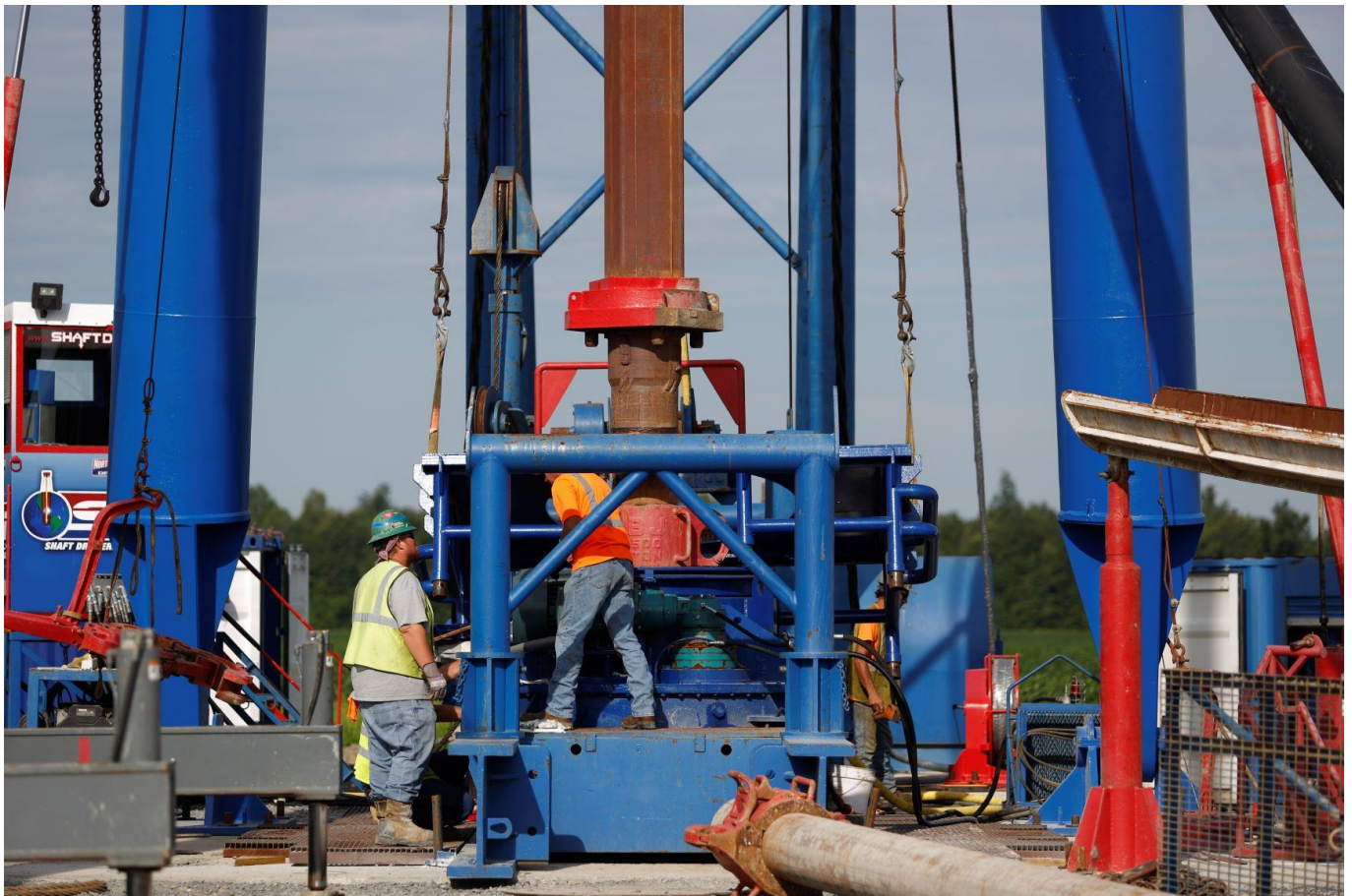
Figure 2: Drilling the shaft pilot holes at Poplar Grove
