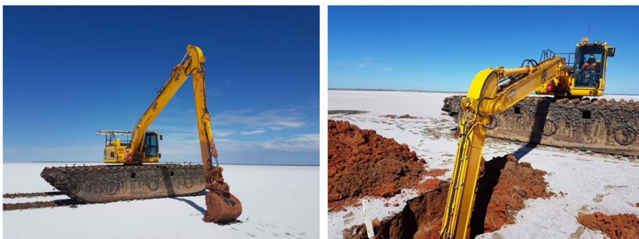
Figure 13: Excavation Activities at Lake Irwin
