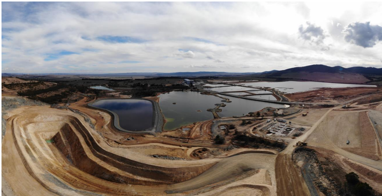
Figure 8: Completed box cut and foundations for the paste plant.
