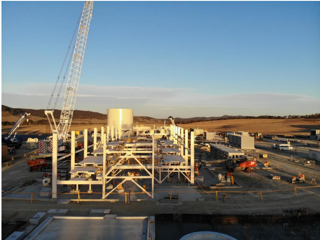
Figure 4: Flotation building – first floor structural steelwork.
