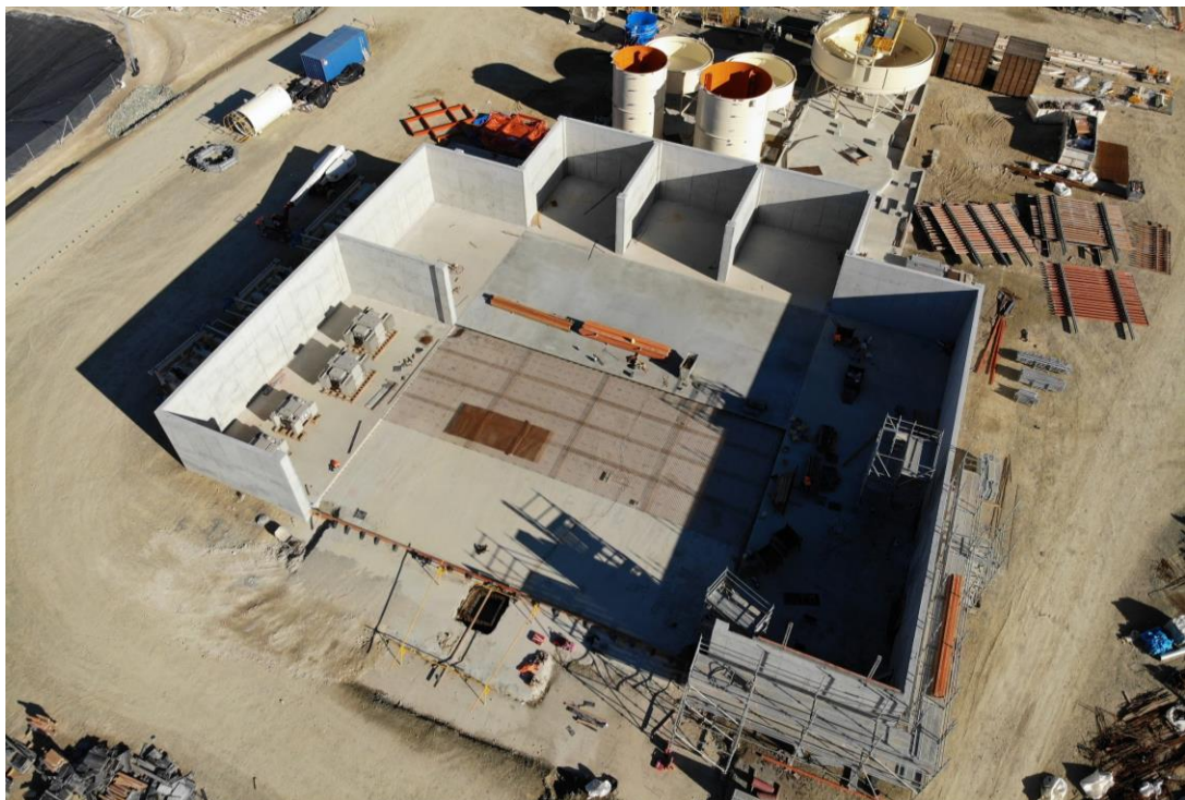
Figure 5: Concentrate handling area.
