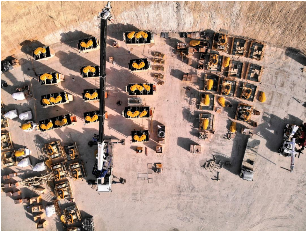
Figure 6: Flotation tanks stored on the ROM pad ready for installation.
