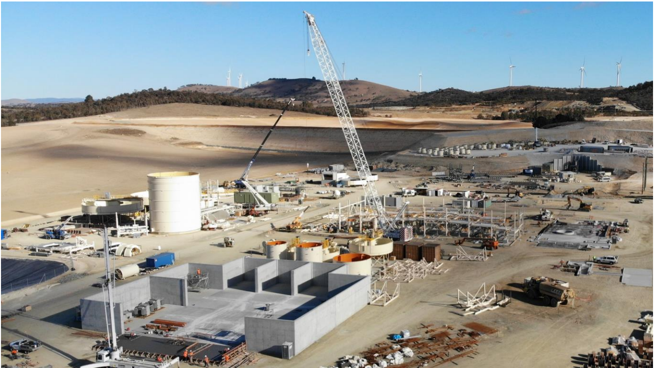
Figure 2: Woodlawn construction site.
