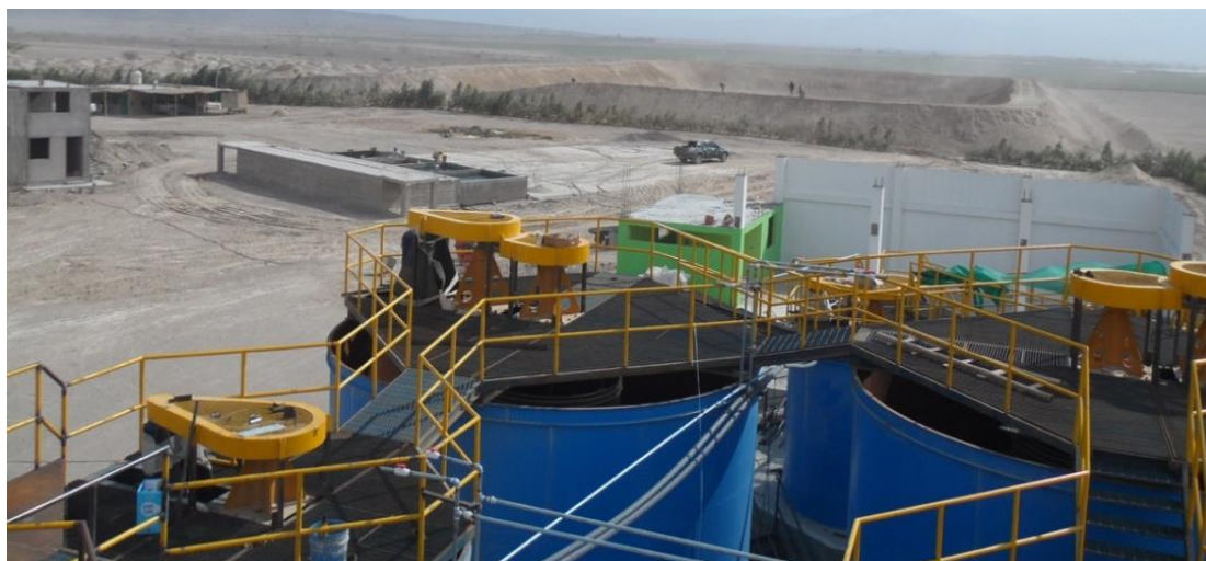
Figure 3 | Vista Carbon & Leaching Tanks, with Tailings Dam in the distance.
